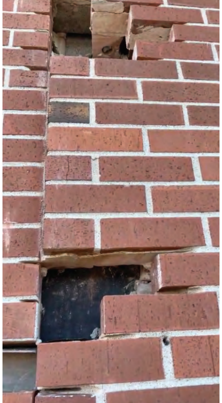
12. Removed brick sections.
