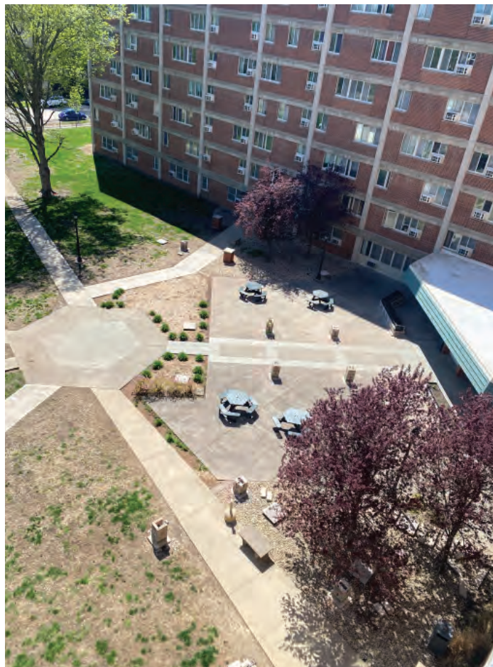
12. Progress of brick piers and planters.
