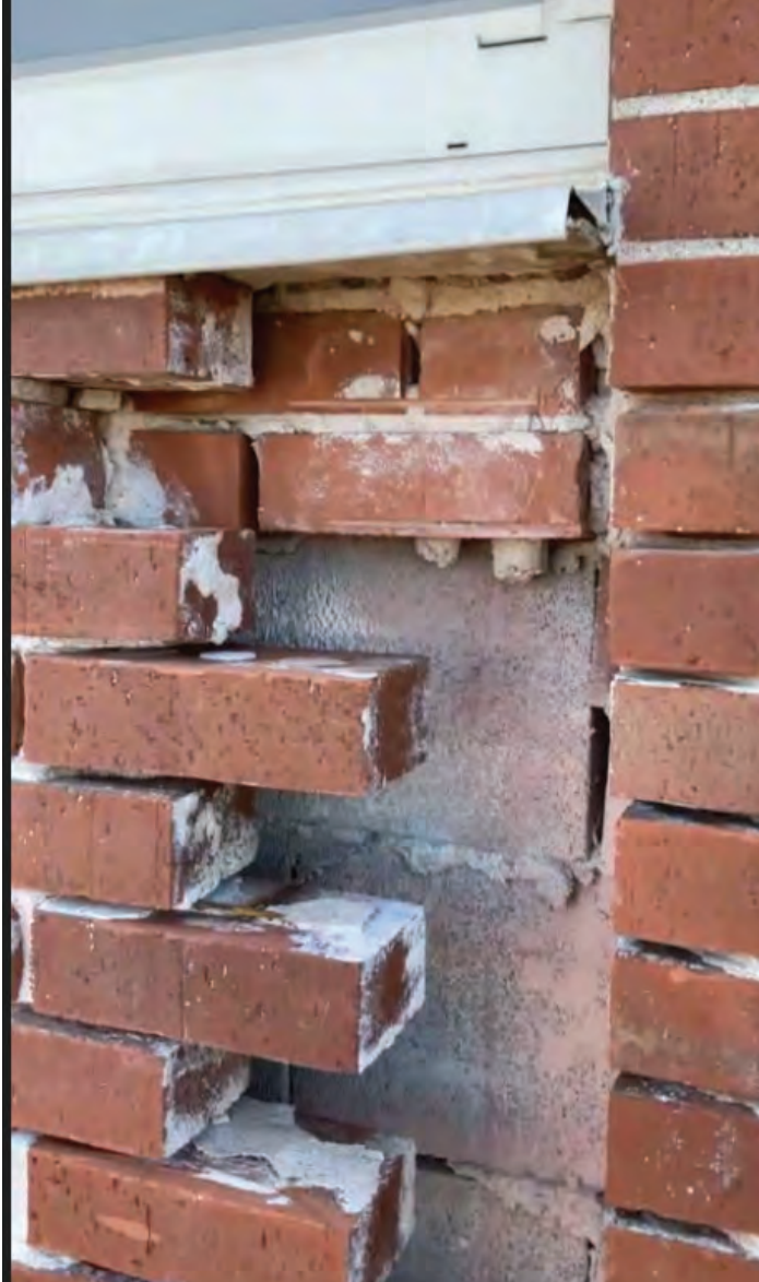
1. Opening above lintel showing second layer of brick below window.
