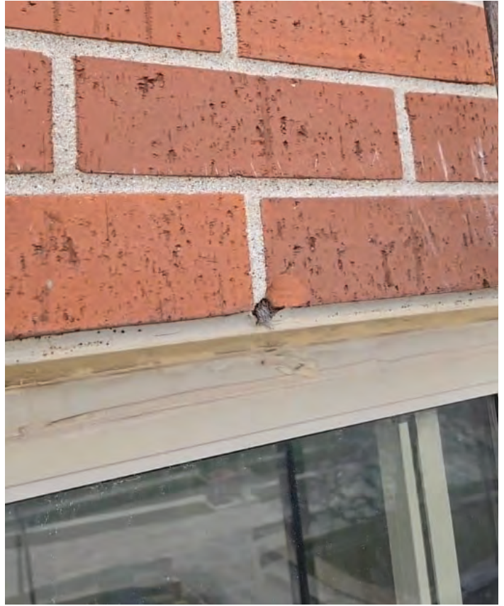
10. Weep holes with steel wool above lintels.
