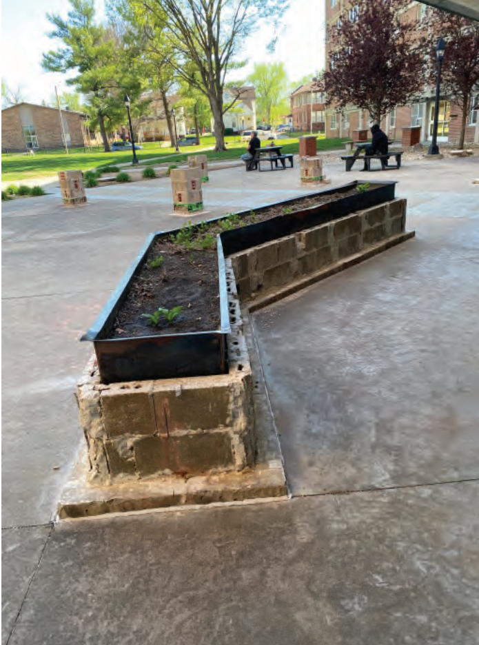
13. All brick removed from most piers and both planters.
