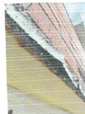
Lintel corrosion
