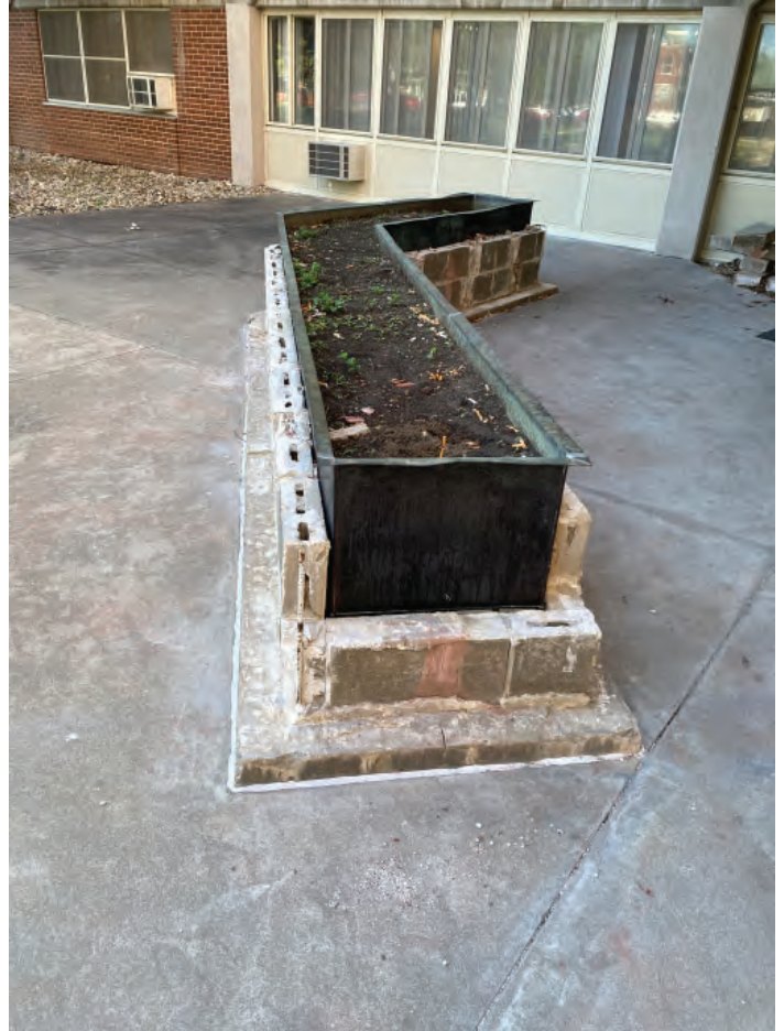
14. All brick and some CMU block removed from the planters.
