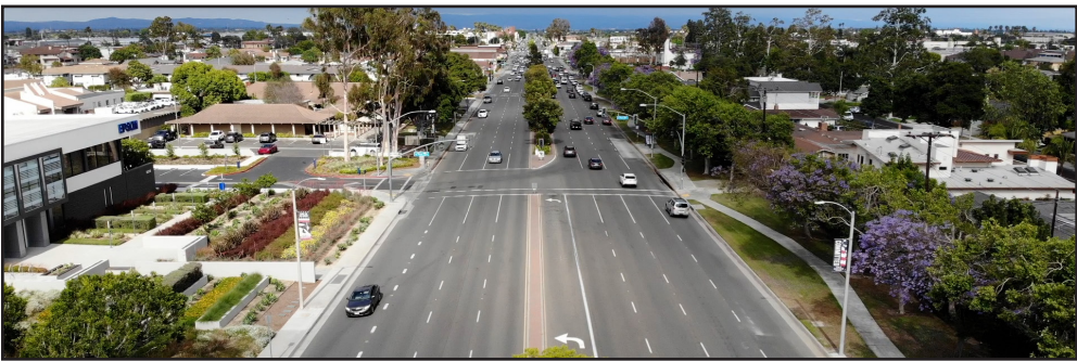
An overhead view of Katella Ave. next to the Los Alamitos Civic Center facing away from the 605 Freeway.
