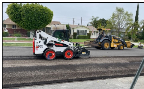
An example of the grind and overlay process mid-construction.
