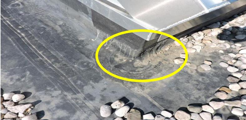
2). At the rear and near a few of the HVAC units there were noted **screws and debris mixed in with the rocks.** It these locations a strong magnet
