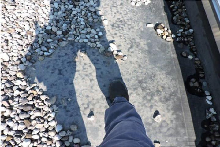
**3). There is loose underlayment on the roof next to the rear left skylight.** The underlayment is buckled upward in this area. Re-secure this area is advised.
