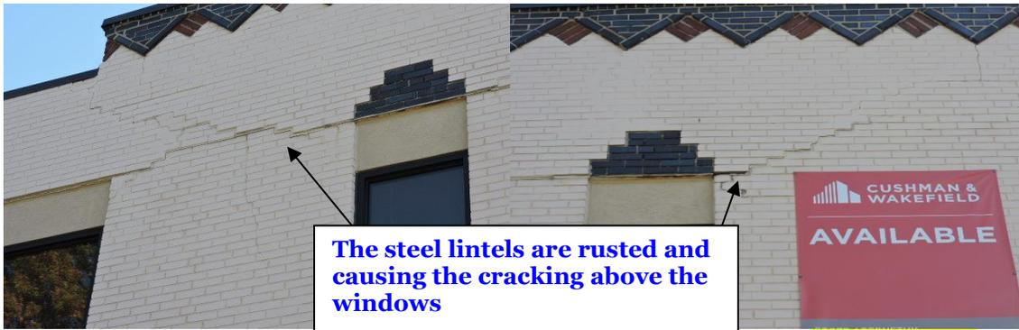
The steel lintels are rusted and causing the cracking above the windows
