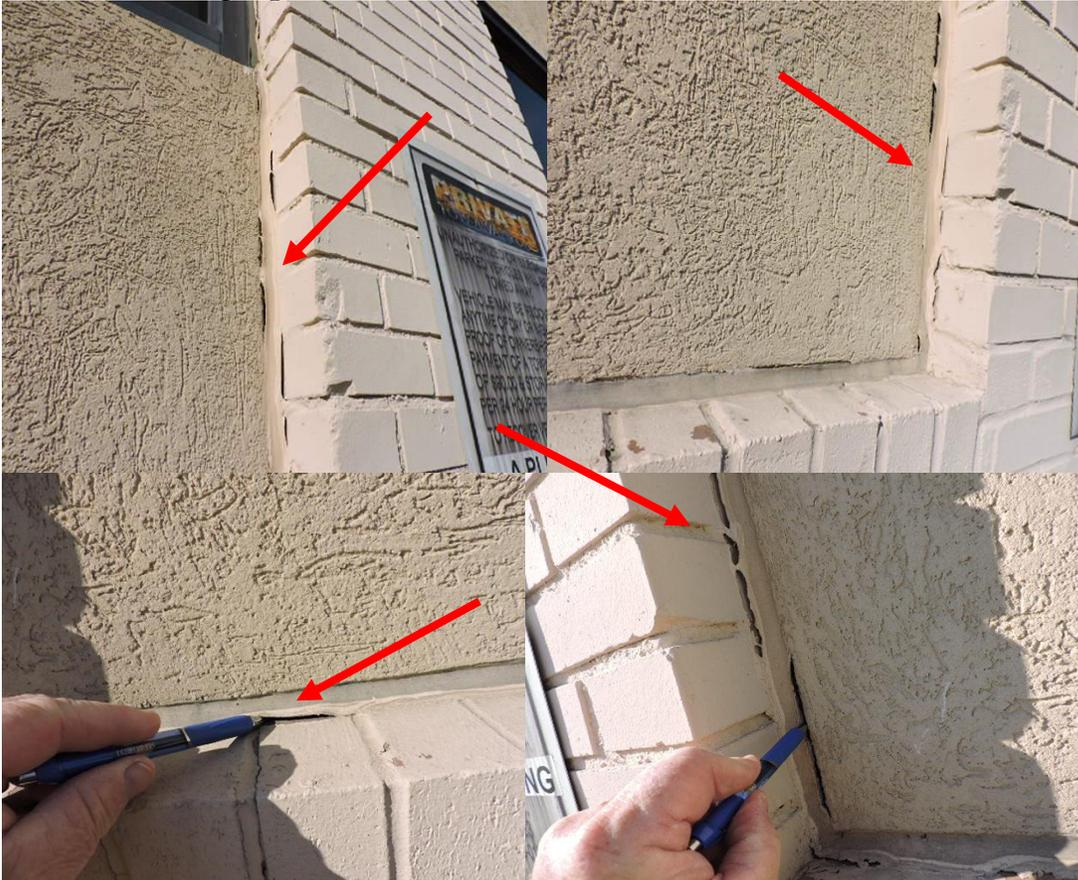
The EIFS appears to be in good condition on the wall surfaces and there are only a few dents and impact cracks in the finish. These can be easily repaired and re-coated. The EIFS poses no issues at this time.
