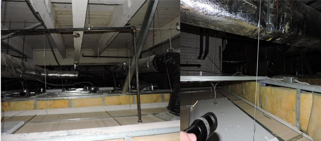
The stains are on the rear roof deck of the area above the break room/kitchen are more concerning. It appears that the lower EPDM roof has leaked in the past near the drain system that is in the center of the lower roof. The movement of the rock ballast was not attempted by the inspector but this may need to be done for a more exhaustive inspection of that lower rear roof.
