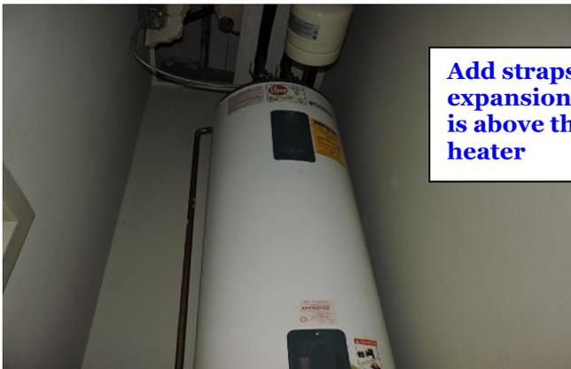
Add straps to the expansion tank that is above the water heater
