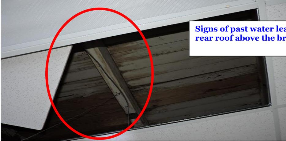
Signs of past water leaking at the rear roof above the break area
