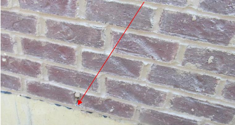
**7). Brick/Window installation** - Expansion gaps between the stone mortar and the window frames are needed. If the brick is too tight against the window frame, there will be excess stress placed on the window frame by the expansion and contraction of the brick and mortar, and also then from distortion of the window frame joints where the top and bottom of the window side jambs intersect the head and sills.
