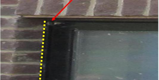
**8). Weep Holes at Window Sills -** This window sill was installed with stone. This is an excellent material because it is one continuous piece and there are no gaps that can take on water. A 15-degree slope is the best slope to have for the stone sills so that water can drain away from the window frame surfaces.
