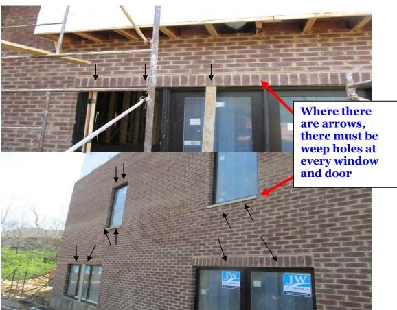
In 2018, the requirement for weep holes had increased from simply installed at the bottom of the stone or brick at the first course of the brick or stone to several other locations. Now, at the top of every door and window, there must be a weep hole for drainage. They also must be installed at gable walls where the bottom of the gable touches the top of the wall plate. There may be other locations as well; local building codes vary in what is adopted from the national building code requirements.
