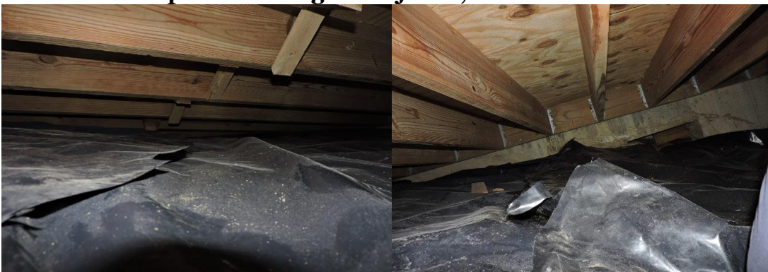
Far left crawlspace showing clean joists, no mold
