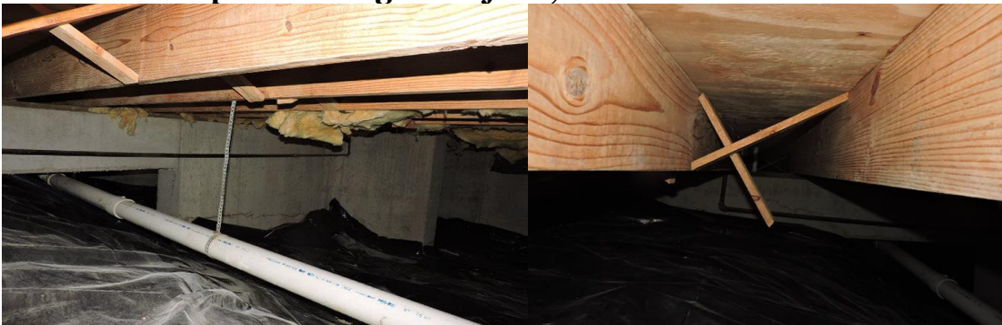
Center Crawlspace showing clean joist, no mold.
