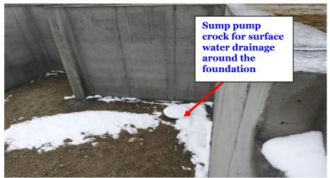
The wall ties had been removed from the wall surfaces and patched on the exterior wall surfaces. The foundation is straight and noted with no leaning or deviations from plumb.
