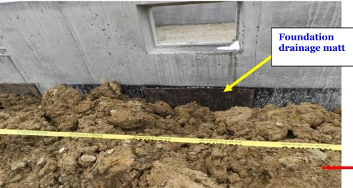
**2).** There was a concrete cast-in-place **foundation** installed on the site. It was noted to be plumb and square. With all the offsets in the foundation no calculations were attempted to determine the exact foundation conditions as in comparison to the drawings.
