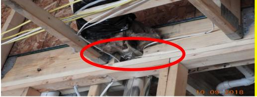
\*\*11). Nail all floor joists that overhand the beam in the basement. Any joist that extends past the beam by more than 3" must be nailed off so that it will not cause floor noise in the future
