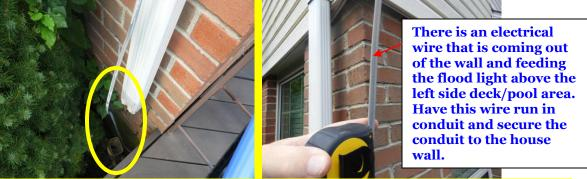
7). At the corner trim of the upper siding, there is some EPS foam that has slipped down out of the corner trim. Have the foam re-secured into the corner trim section. Repair the damaged downspout below the corner trim on the rear right house corner
