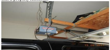
**a).** There is a **loft constructed using the garage door opener brackets as supports**. Because these brackets are attached to the bottom cords of the truss system and the trusses are not intended to support any additional imposed load other than that of the truss members, the disassembly of the loft is advised.
