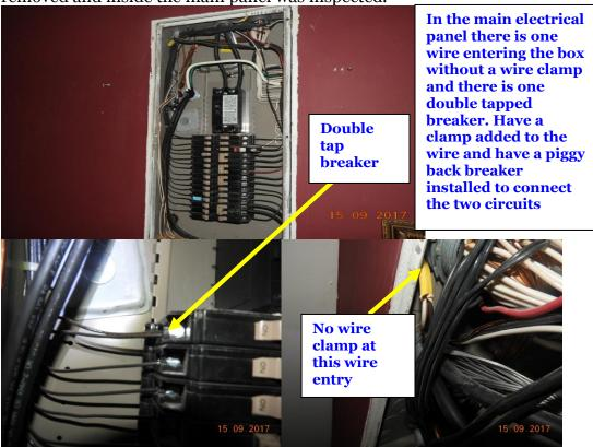
There were no major observed errors in the wiring technique. No water access was observed and the circuits showed no evidence of overload or overheating.
