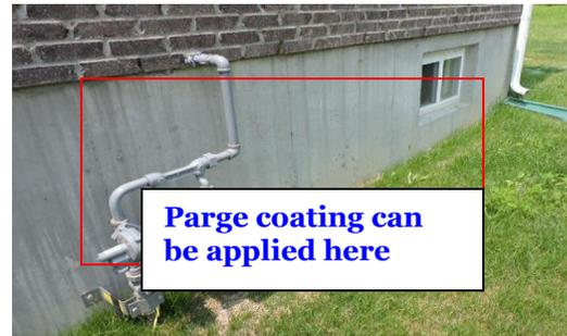
**7).** The application of a **parge coating** to the surface of the exposed foundation on the left, right and rear of the home was recommended. There is a direct coat system that can be applied to the concrete surfaces in all these locations. It is A good sealant which makes the foundation much more attractive.
