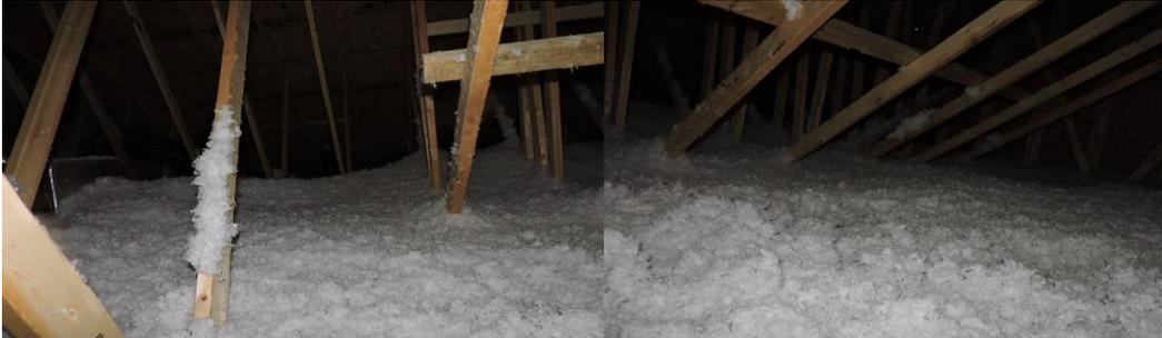
30). The **venting** of the upper attic appears to be sufficient at the apex of the attic space and at the soffit areas. The air passages at the attic areas near the truss bearing points were clear of insulation and blockage. The air passages had baffles installed at the soffit area of the attic.
