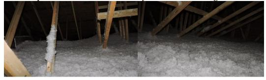
**30).** The **venting** of the upper attic appears to be sufficient at the apex of the attic space and at the soffit areas. The air passages at the attic areas near the truss bearing points were clear of insulation and blockage. The air passages had baffles installed at the soffit area of the attic.
