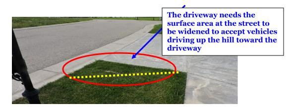
17). The concrete **driveway surface** is in good condition. Use a water sealant on the surfaces in the future is suggested. The application of Weather X or Enviro Seal is recommended because these are durable products. The best application is with a thick roller and a rolling pan. Be careful with application. Some types of sealants if they are not applied properly can turn color and make the concrete discolored. Obtain as much information on the product application as possible.
