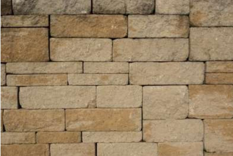
**Some of the ACMV is applied tightly at all joints with no mortar observed. Some is installed with gaps in the stones with mortar between the stones so that they appear to be similar to a real mined stone. All are adhered to the scratch coat and then “stuck” against the scratch coat with N type mortar.**
