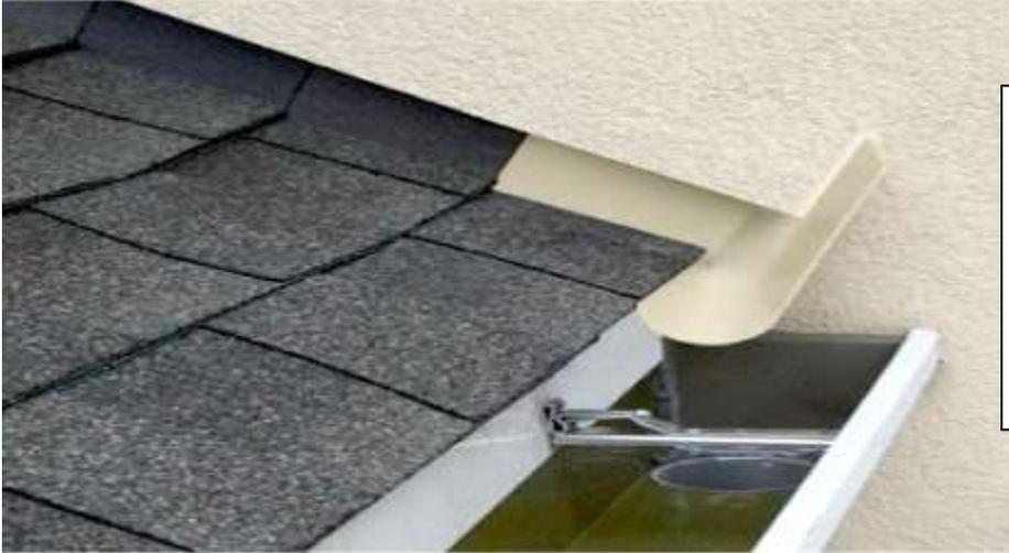
**While the pictured diverter is installed in an EIFS system, the same diverter would be installed with ACMV stone**
