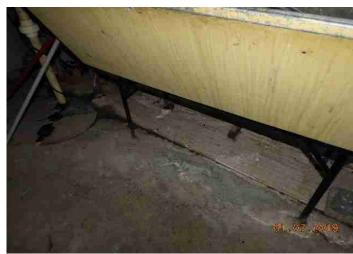
There is mold in this basement due to water leaking into the basement on the center wall. The conditions are encouraging mold growth to propagate. Have the wall material removed.
