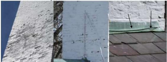
b). The center chimney needs to have the base flashing sealed at the bottom of the chimney surface where it intersects with the slate.
