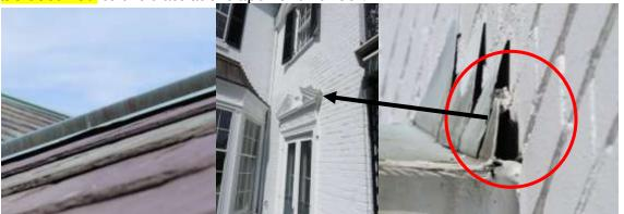
i). The **flashing above the rear door** to the house needs to be secured back into place.
