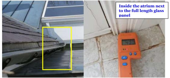
f). Most of the **gutters** were noted to be installed properly with proper pitch to the downspouts in most locations. There needs to be adjustment of the front left gutter above the center of the left of the home and the rear left gutter on the same, lefthand side of the home. At each location the gutter is bowed downward and is not draining and there is water overflow at that location.
