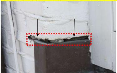
d). On the rear of the home, the left side gable wall has a counter flashing that needs to be re-secured into the mortar where it has pulled out at this time.
