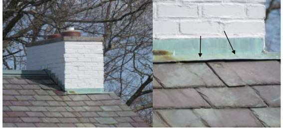
c). There is a **counter flashing** above the rear most right side door that **needs** to be secured and mortar tucked into the rivulet
