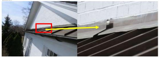
e). The front face of the home, where it connects to the \_\_\_\_\_needs to be re-flashed and the gutter needs to be corrected. There is active water leaking at the intersection of the left atrium wall and the front wall of the addition
