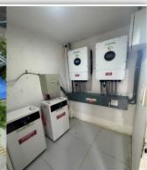
40kW On-Grid Inverter w/ 40kWp PV System Nakutan Extension, Marikina City
