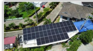
24kW Hybrid Inverter with 31.9kWp Solar PV System The Entrance of The Woodlands Resort, Uloan, Cebu
