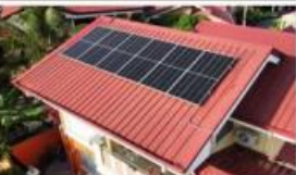
5KW Hybrid solar power system Liloan City
