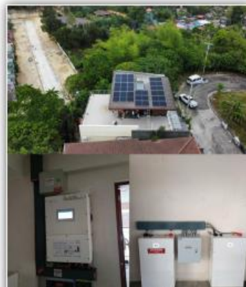
6kW Solis Hybrid Inverter w/ 5.5kWp Solar Panel & 10.24kWh BESS Talaman, Cebu
