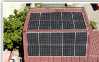
6kW Solis Hybrid Inverter w/ 5.5kWp Solar Panel & 10.24kWh BESS Talaman, Cebu
