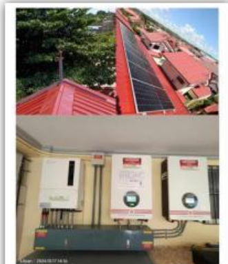
6kW Solis Hybrid Inverter w/ 5.5kWp Solar Panel & 20.48kWh BESS Eastland Estate, Yalk-Lilean, Cebu
