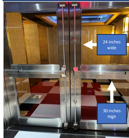
Glass Doors into South Ballroom Looking Out 30 inches High X 24 inches wide
