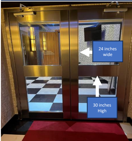
Glass Doors into South Ballroom From top of Staircase from Hotel Lobby 4 panels (all same measurements) 30 inches High X 24 inches wide
