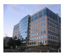
building. The Class A office building includes a six-level parking structure connected by a pedestrian bridge. Miyamoto used slotted web moment connections in its lateral-load resisting system to reduce steel tonnage while providing improved moment-frame performance.
