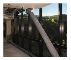
also be deployed in civilian building projects. Miyamoto engineers successfully implemented this high performance technology into the office building, significantly improving performance during a seismic event. Thirty six-inch cylinder-like dampers were strategically installed at the second and third floors.
