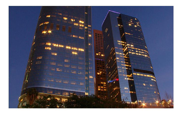
California Plaza is a mixed-use office/ retail/entertainment complex constructed on a steep hillside atop Bunker Hill downtown Los Angeles. MHI performed preliminary design of the two office towers, which feature steel perimeter tube frames and final design for the Plaza, featuring fountains, reflecting pools, an outdoor ampitheater, bridge and funicular railway, subterranean parking structure and the adjacent Museum of Contemporary Art.
