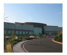
Miyamoto provided design for construction of the "Waste Connections" office headquarters in Folsom. This building is a threestory, non-bearing, tilt-up concrete structure used for Class A office space. The second and third floors are constructed with concrete fill over metal deck supported by steel wide flange beams. This composite floor
