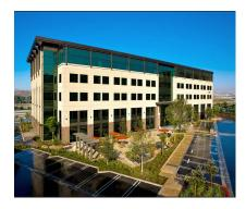
is visible from the 5 freeway, and positioned at the entry of Newhall Ranch, a master planned community of 21,000 homes. The facility uses slotted-web steel moment connections in its lateral force resisting system to reduce overall steel tonnage while improving building performance. The building features 28,000 square foot floor plates, first-class common areas, plenty of light and natural finishes.
