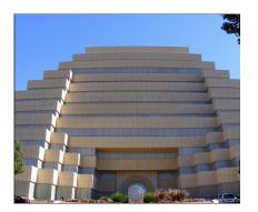
This 11-story, pyramid-shaped mission-critical building is the Headquarters of the Department of General Services and became one of the first buildings in the United States to use seismic dampers. The structural system uses steel special moment resisting frames with fluid viscous dampers (FVD) to offer an elastic response to earthquakes and to avoid business disruption after earthquakes.
