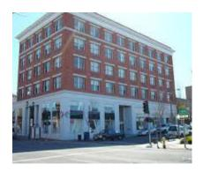
Built in 1917, the Professional Building stands as one of the largest buildings in downtown Eureka. Located in an earthquake vulnerable area with poor soil conditions, this unreinforced masonry building was in need of a seismic rehabilitation. Using performance-based engineering, the existing interior steel gravity frames were augmented with new slotted bolted friction dampers, adding
