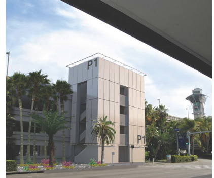
LAX Parking Garage and Terminal Elevator Replacements Los Angeles, CA
