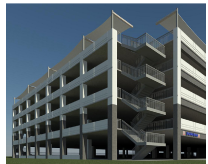
Qualcomm Pacific Center Parking Structure San Diego, CA
