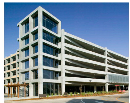
California State University, Sacramento, Parking Structure II Sacramento, CA
