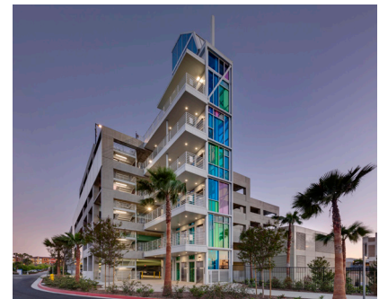
Sharp Chula Vista Parking Structure Chula Vista, CA
