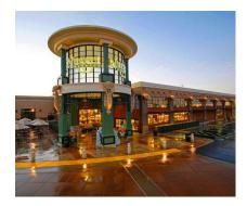
and plywood supported by open web steel joist and girders. The focal point of the market is its grand entrance tower. The glass, wrought iron and concrete sculptures that define the tower are all supported by an ordinary steel moment frames. The exposed concrete slabs on grade are painted, stained and sealed to provide an artisan feel to the home town market
