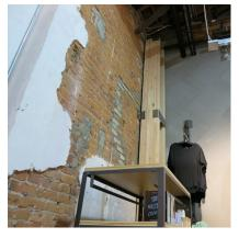
typical steel strongback post to blend with the existing timber components of the original building. Using the retrofit methodology selected, the retail space was able to remain operational during normal business hours and construction was performed in the evening hours to significantly reduce the financial impact of construction to the store.
