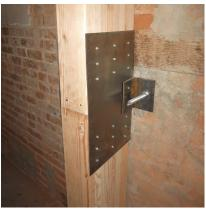
Miyamoto provided structural engineering services to seismically upgrade an existing unreinforced masonry (URM) structure to be in compliance with the City of Santa Monica building code. A series of strongback posts and wall anchors were installed on the interior wall faces to reduce the potential of out-of-plane collapse in an earthquake. Glulam posts were selected in lieu of the
