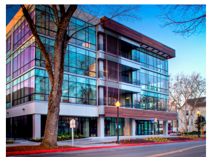
2600 Capitol Office Building, Sacramento, CA
