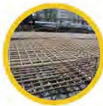
solid foundation with composite rebar
