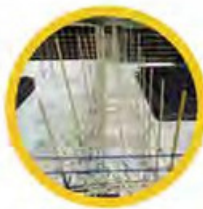
the walls of the frame composite rebar
