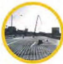
experimental foundation work using composite rebar
