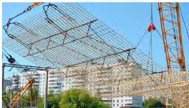
The use composite rebar for waterproofing roofs
