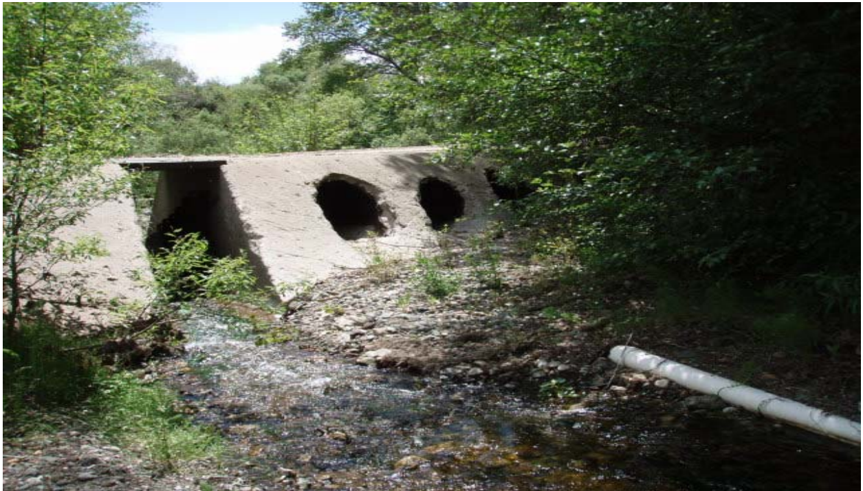
Figure 15. Looking downstream to Ferrasci Road crossing, Santa Rosa Creek
