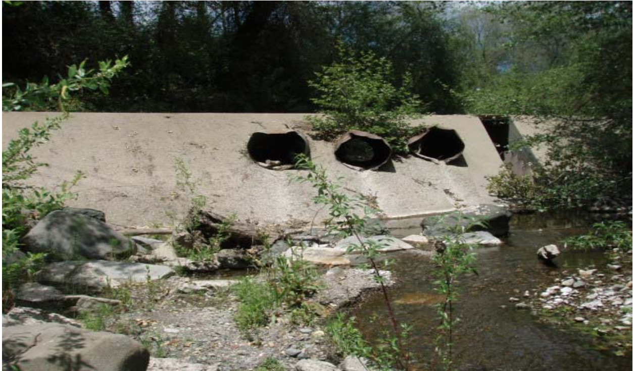
Figure 14. Looking upstream to Ferrasci Road crossing, Santa Rosa Creek.
