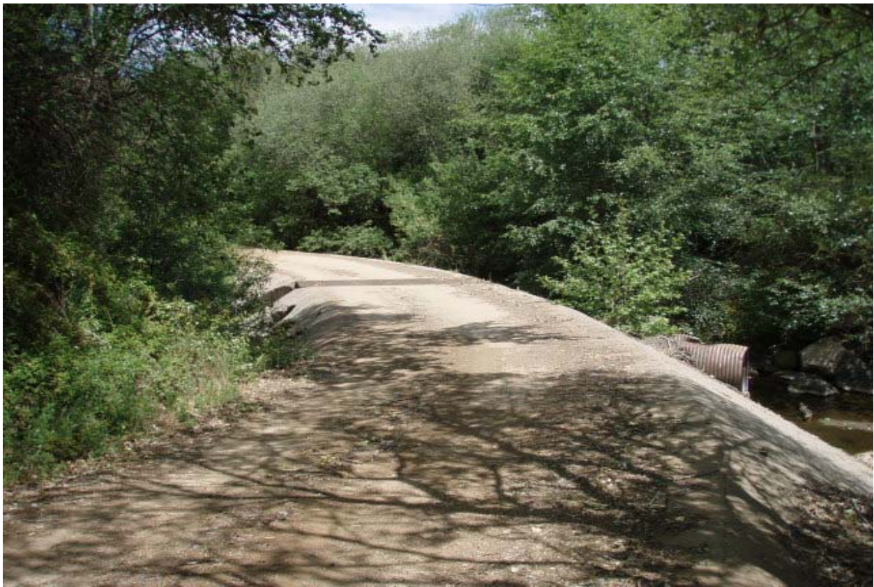
Figure 13. Ferrasci Road crossing at stream mile 3.4.
