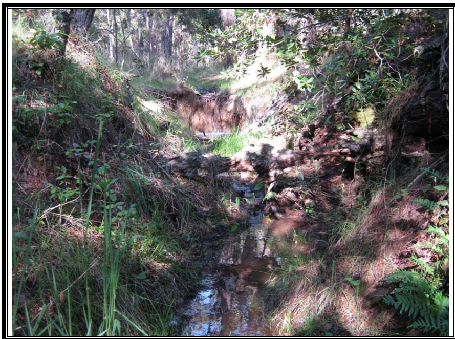
Figure 9. Incised area downstream of the active headcut.
