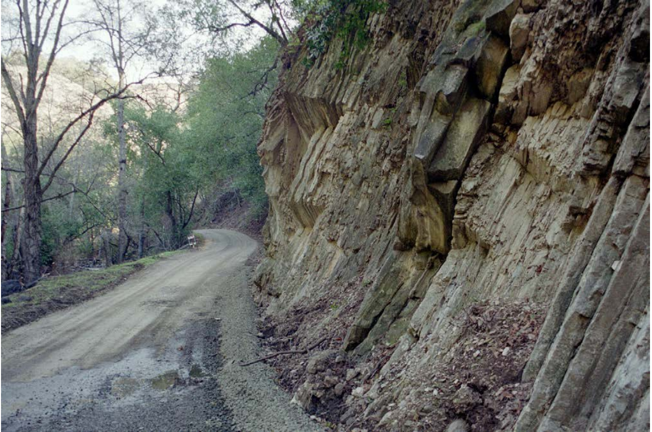
Oceanic Fault - located just outside the District on Santa Rosa Creek Road
