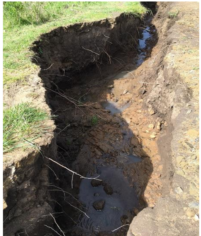
Trail Erosion at Harmony Headlands Photo: Connie Gannon
