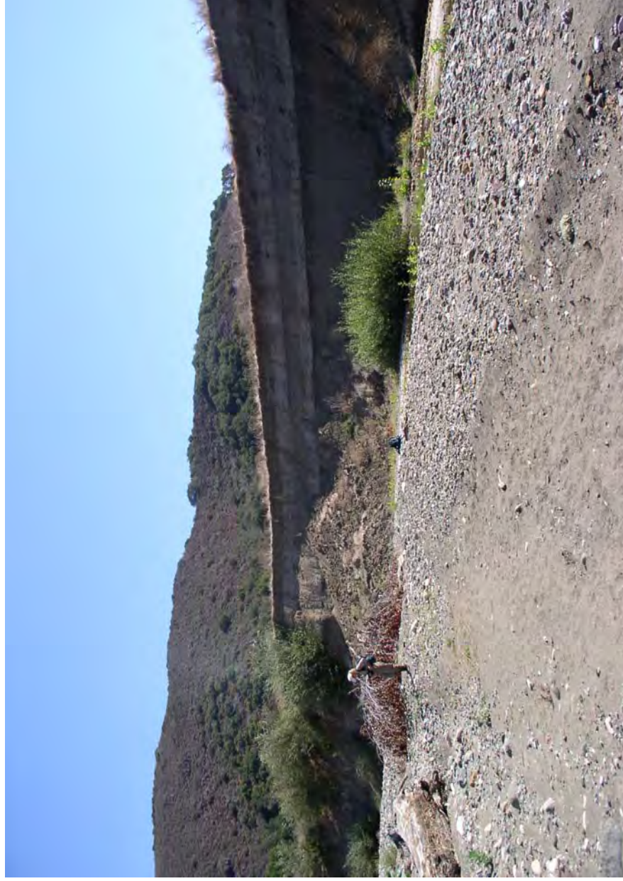
Figure 12. A portion of the dry section in Santa Rosa Creek, 2005.
