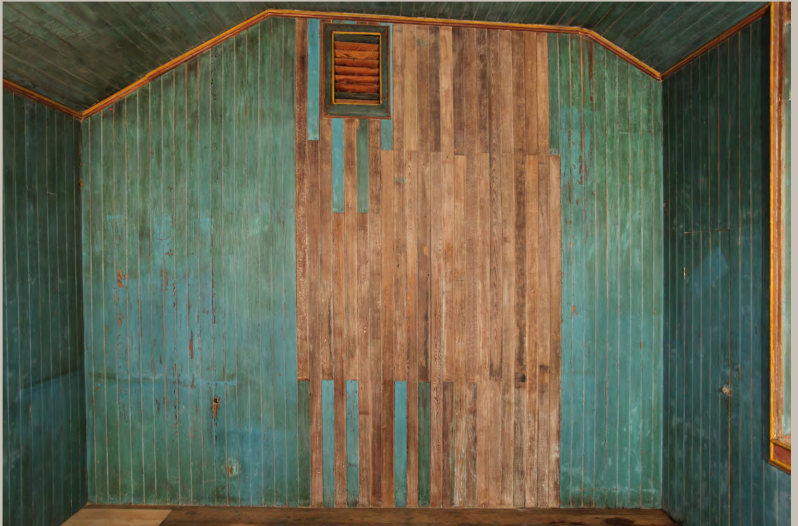
The south wall prior to restoration
