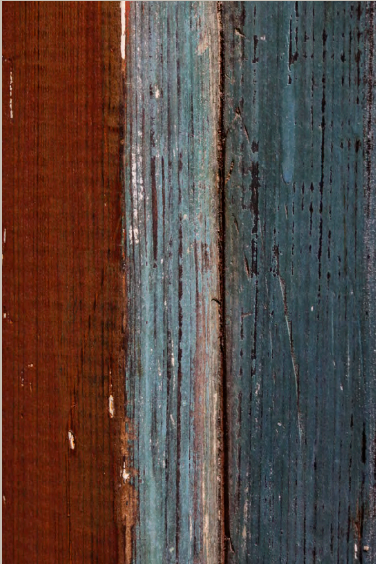
Detail of the entrance door showing the original blue paint on the side of the casing
