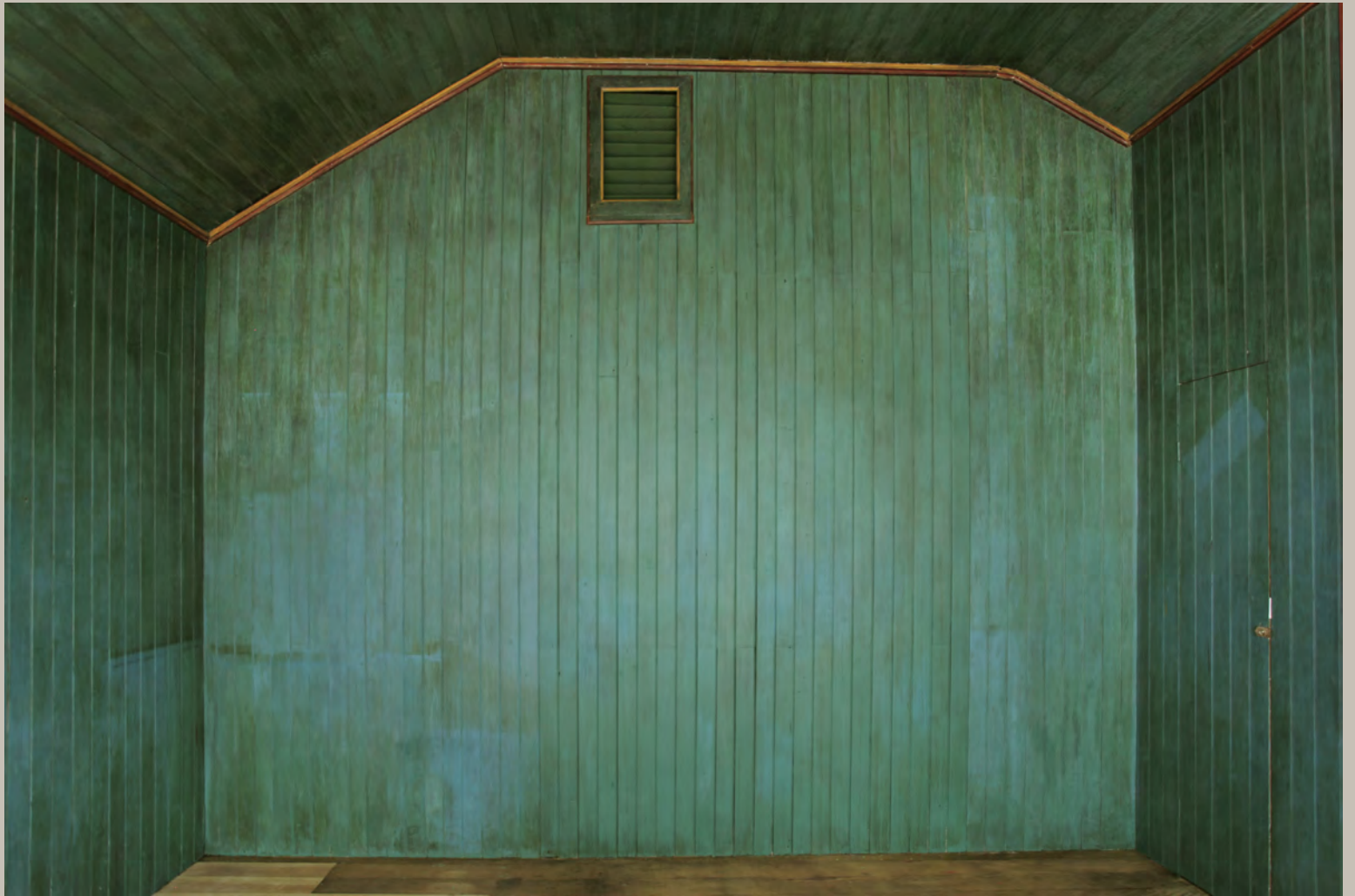
The south wall after restoration
