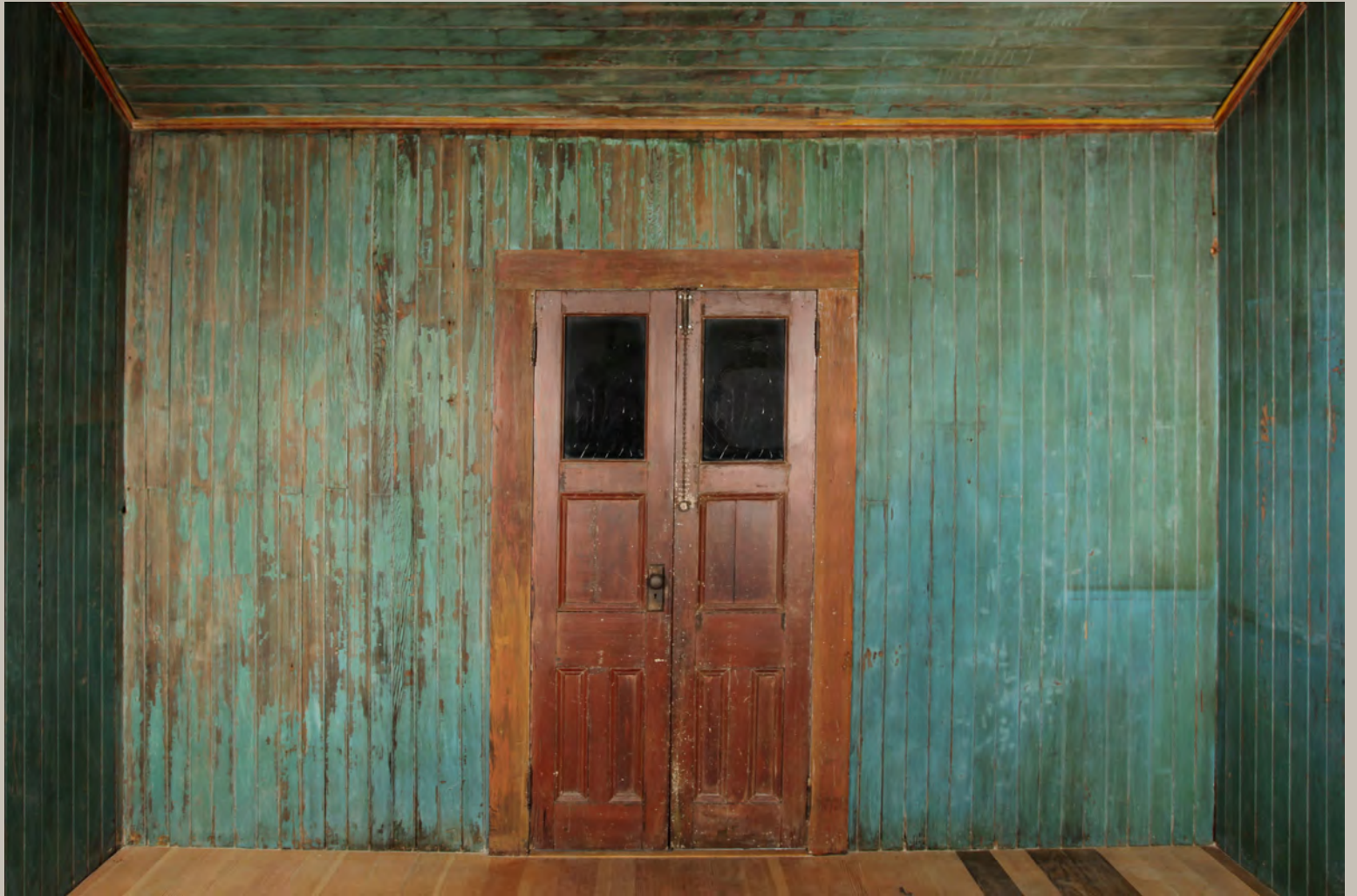
The east wall prior to restoration
