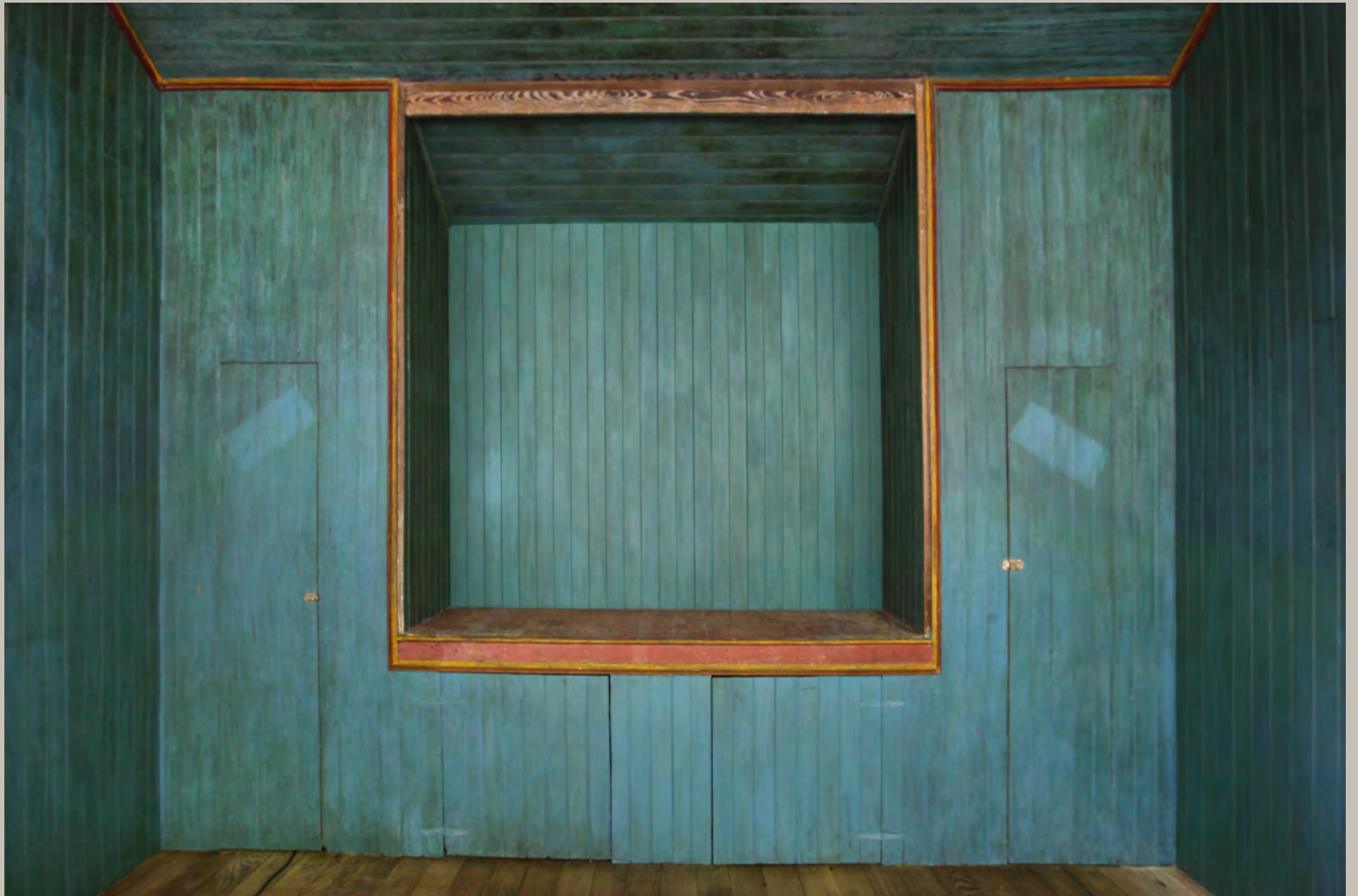
The west wall after restoration
