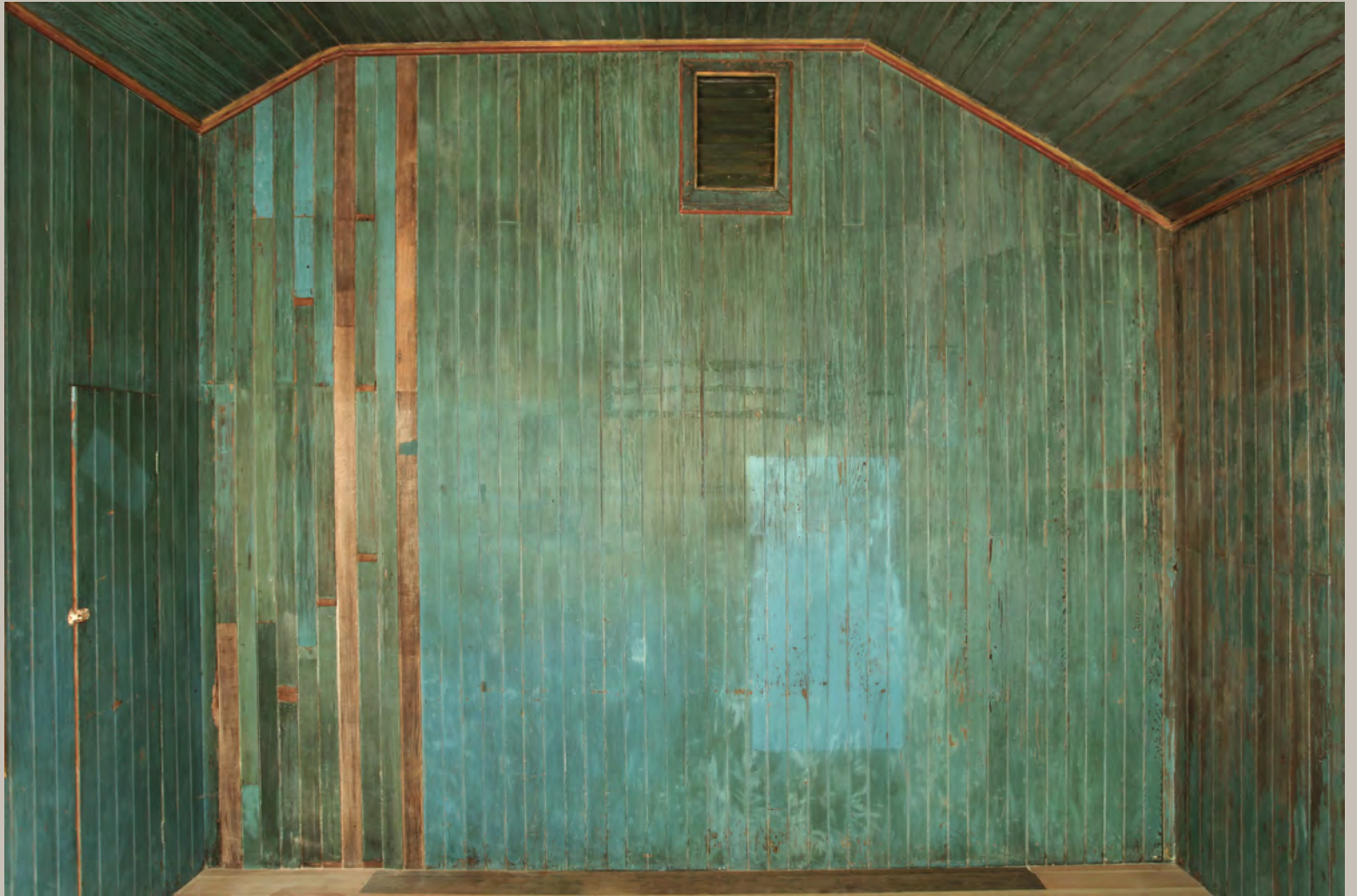
The north wall prior to restoration
