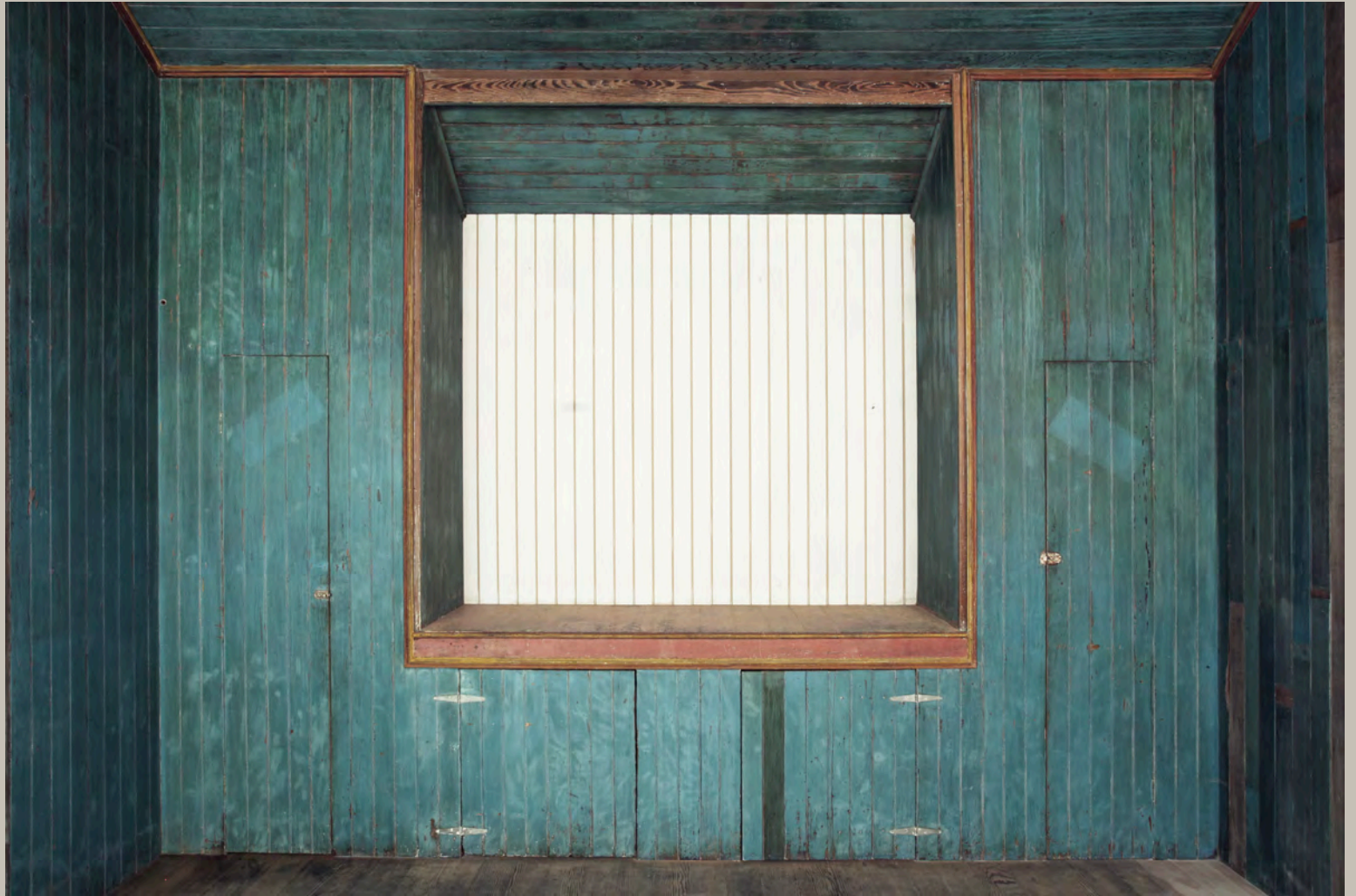
The west wall prior to restoration
