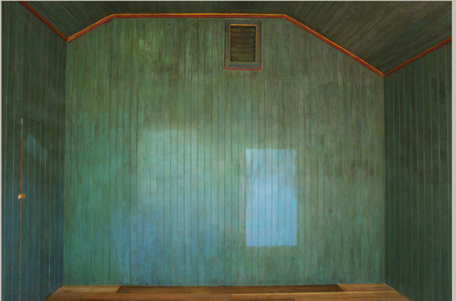
The north wall after restoration
