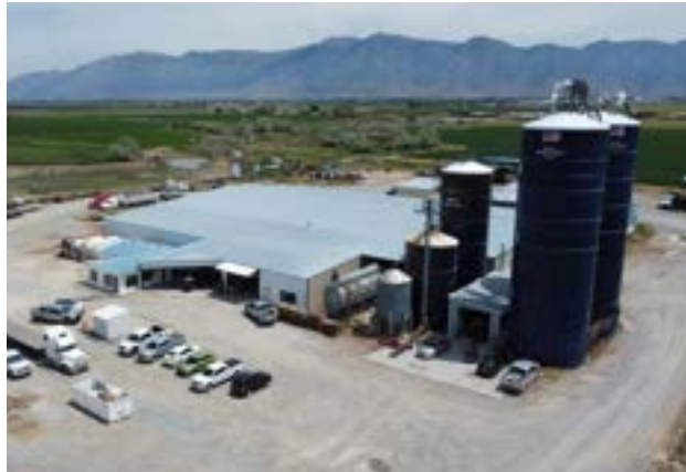
Main Warehouse Located in Corinne Utah
