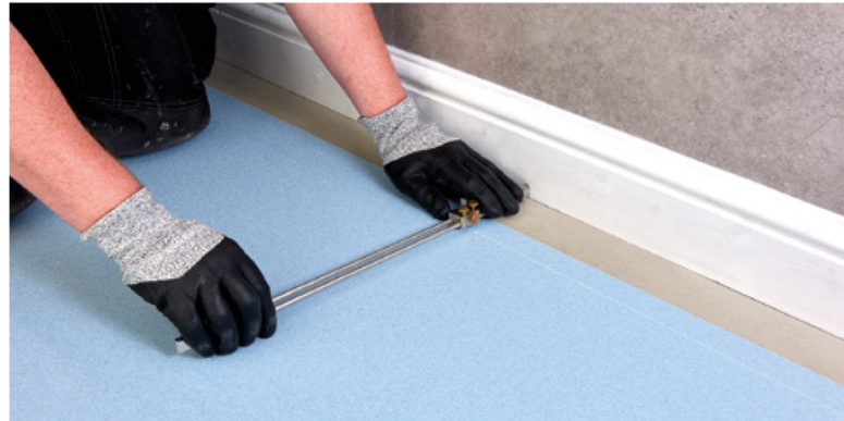
Figure 3.2 Scribing the wall profile
