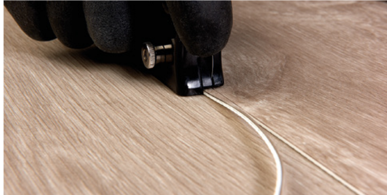
Figure 3.5 Cutting in the seams
