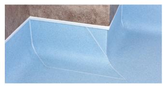
Figure 3.9 External corners 'wrap around method'
