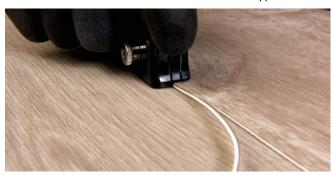
Figure 3.5 Cutting in the seams
