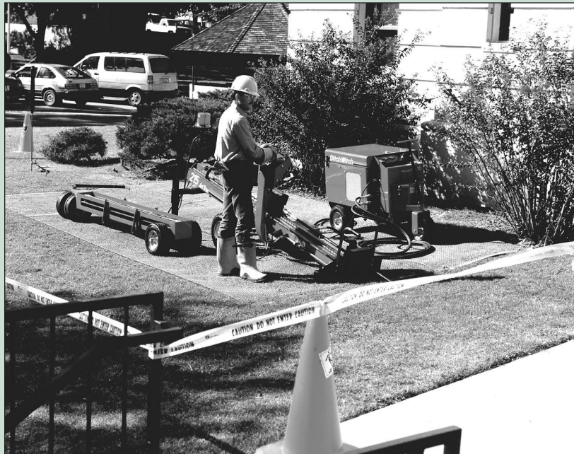
Tunneling equipment involves a cutting tool, connecting rods and/or hoses, a unit that provides thrust or torque, and a field power unit. In some cases, a hand-held locator tracks the cutting head. Operators can make adjustments (“steer”) for both depth and direction as the tunneling proceeds. Accuracy of some methods is within inches of a target (usually an access pit) at the end of the tunneled span.
