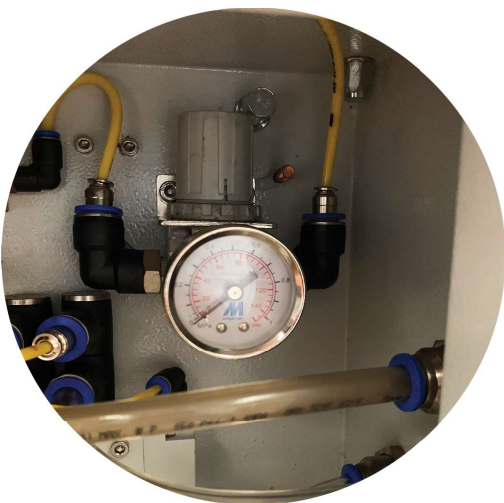
Pneumatic controls pressure gauge with regulator
