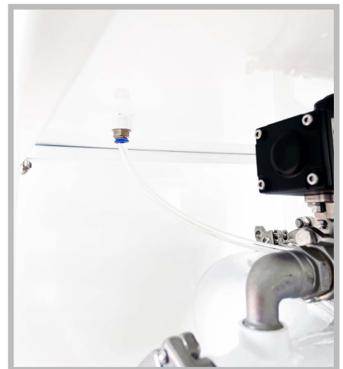
EXHAUST BOX DRAIN LOCATION
