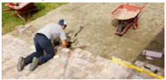
Tamp as if cutting a lawn making lateral then vertical passes. A laser level, especially for larger jobs, is a good choice but string with a line level can also work. When using a mechanical tamper, the machine jumping around a bit will indicate the base is sufficiently compacted. Afterward, bedding (paver or limestone) sand needs to be applied, screed (a straight 2"x4" board) and tamped to a 1" level. Several applications may be necessary. Edge restraints are then installed.
