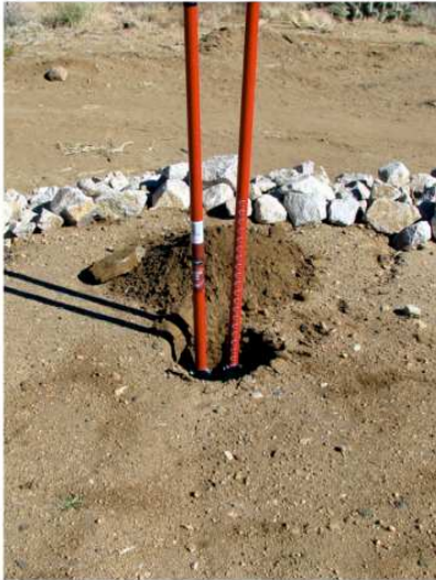
Dig 18-20" deep hole (post-hole digger shown)
