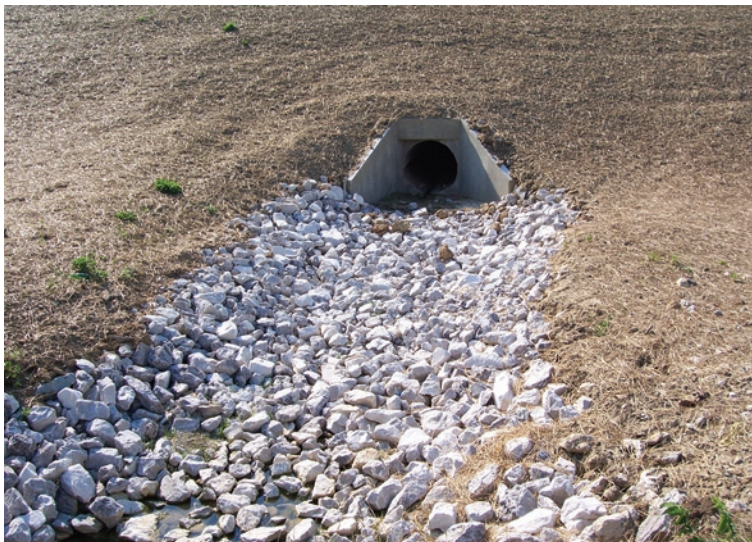
Figure 17. Make sure inlets, outlets, and slopes are well stabilized before leaving the site and filing your "Notice of Termination" for ending permit coverage.
