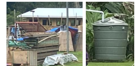
New dormitories being built, new tank, 2025
