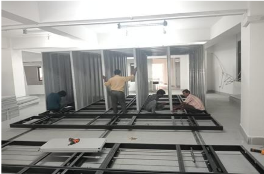
Installation of Compactor Source: Archive Team (July 2024)
