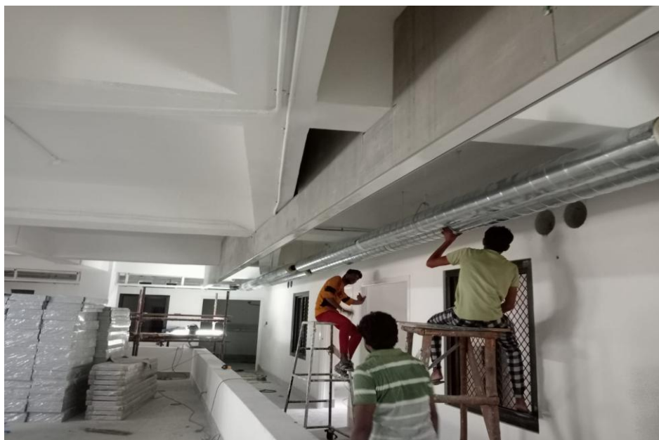
Installation of A/C
