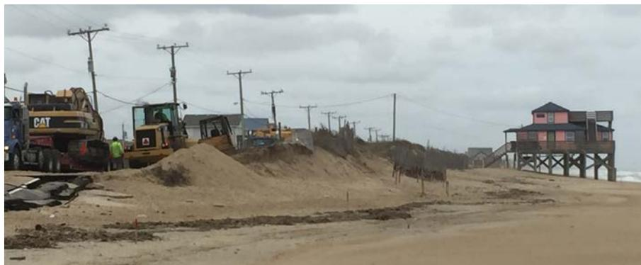
Figure 1: Dunes being bulldozed into place after a coastal storm, Kitty Hawk, NC.
