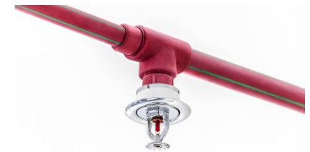
Sprinkler System Check, Test, Inspect
