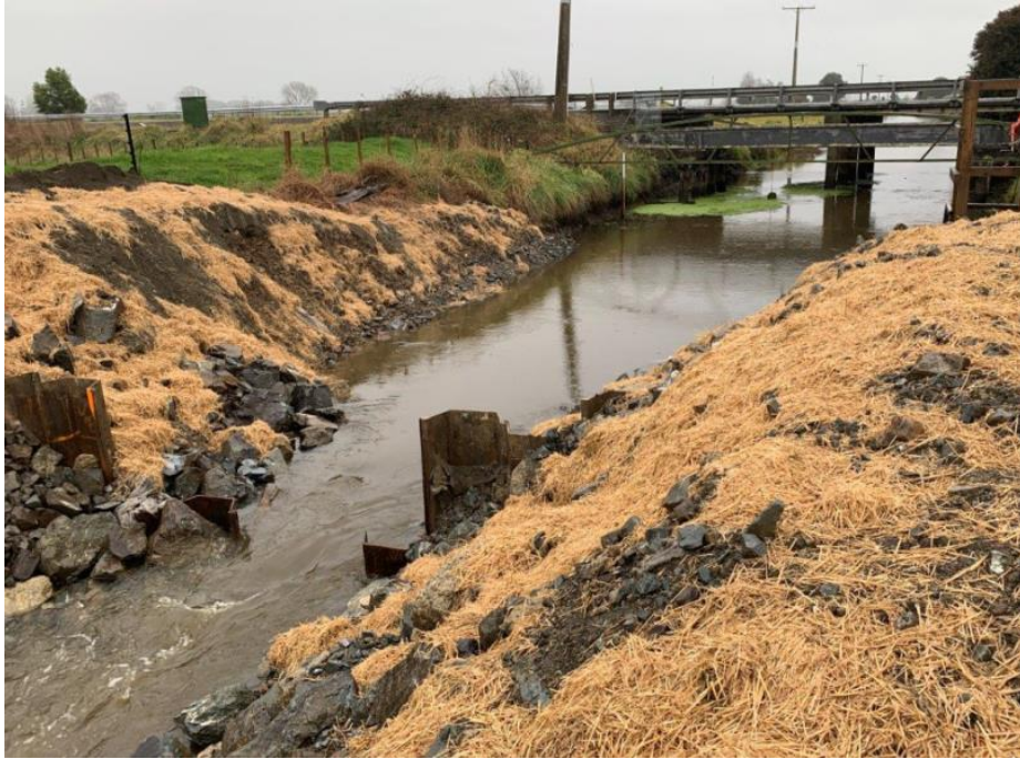
FCS- West modified to prevent sediment transport from W to E and allow drainage
