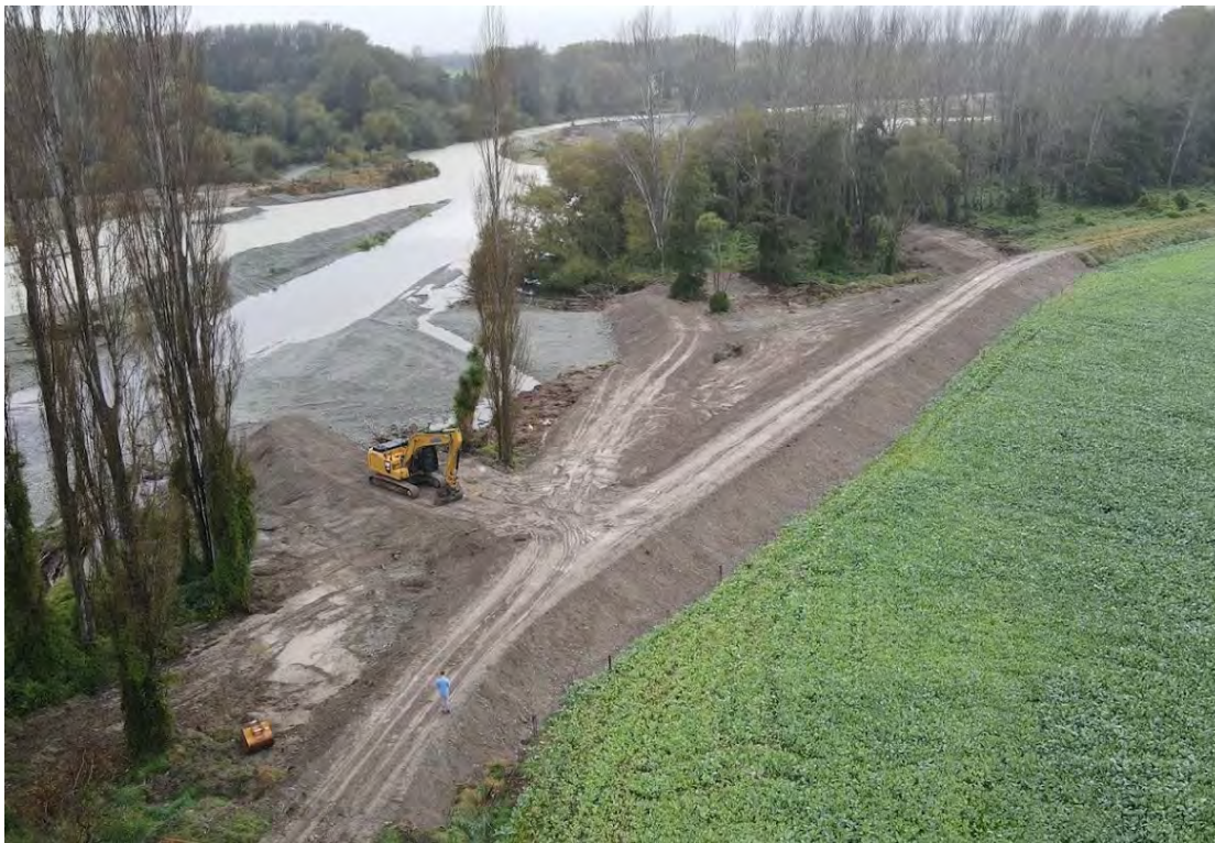
Figure 8-40: Opihi at Collett Rd, following completion of stopbank and erosion protection bund works 23/3/2022.
