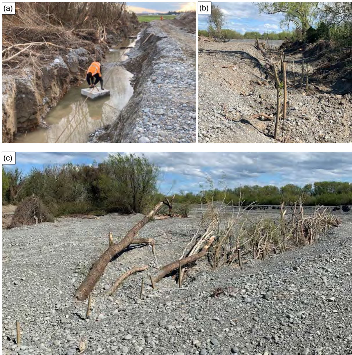
Figure 8-9: South Ashburton at Blacks Road, installation of anchored tree protection at erosion protection bunds: (a) installation of concrete block anchors, (burying willow poles in trench, and (c) completed ATP on upstream edge of erosion protection bund.
