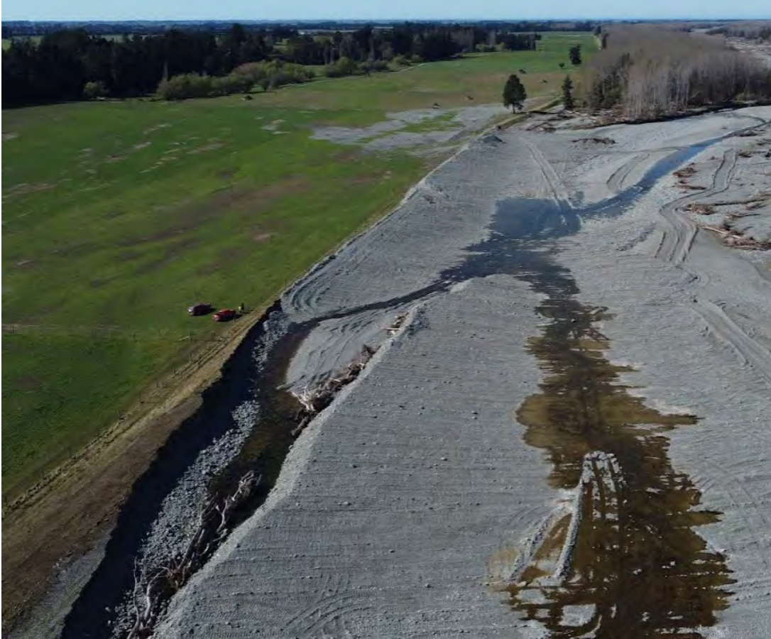
Figure 8-16: Orari at Inglis Rd Site C, looking downstream following temporary work prior to stopbank rebuild, September 2021.
