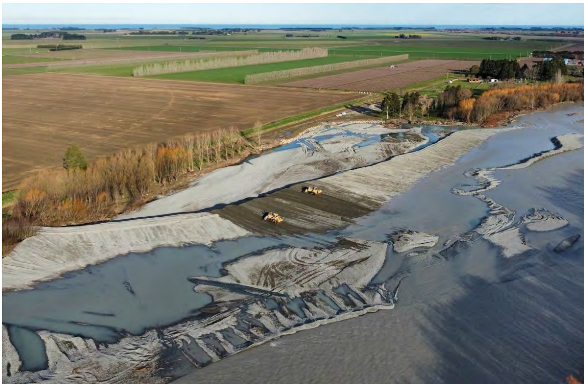
Figure 9-2: Ashburton at River Rd, initial temporary protection bunds, August 2021.
