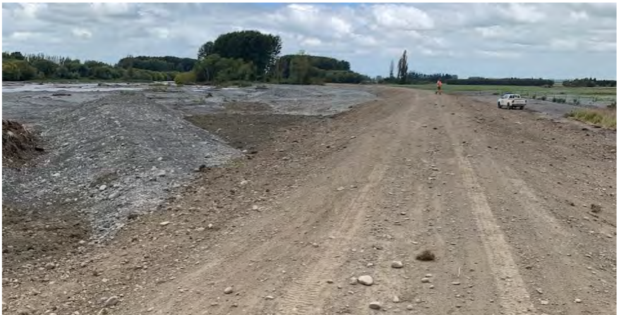
Figure 8-5: North Ashburton at Thompsons Track. Looking downstream from same location as above following completion of stopbank and erosion protection bund repair, 24 February 2022.
