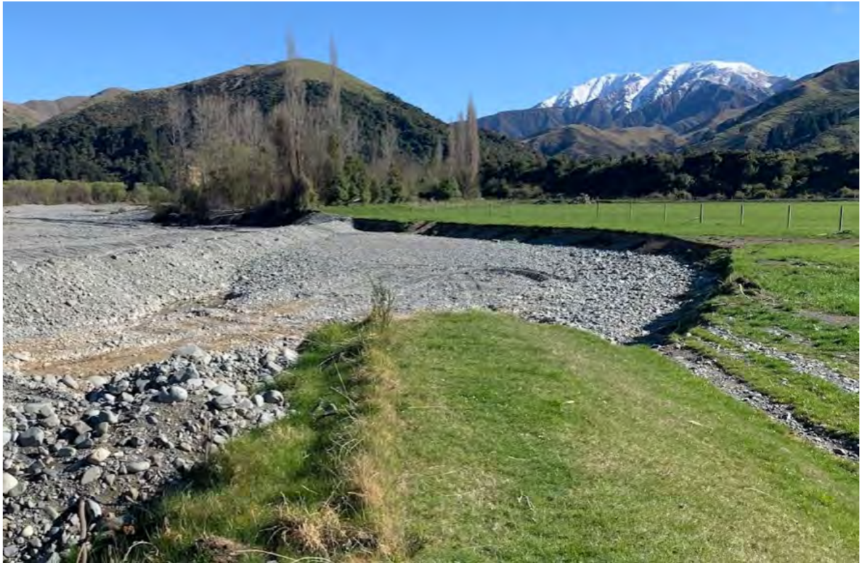
Figure 8-12: Orari at Inglis Rd Site A, Stopbank and edge protection loss - 28/9/2021.
