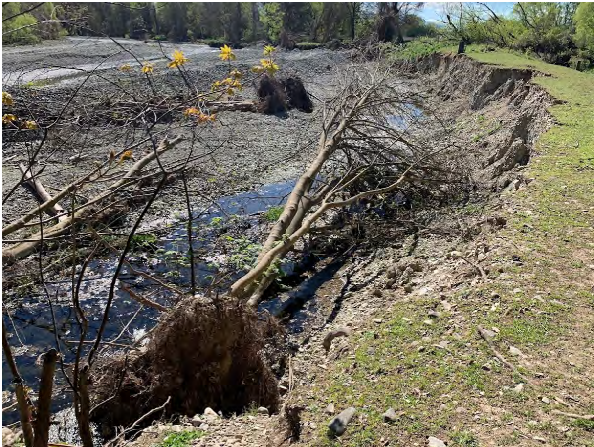
Figure 8-33: Waihi at Hawke Rd Site A, showing flood damage to stopbank 28/9/2021.
