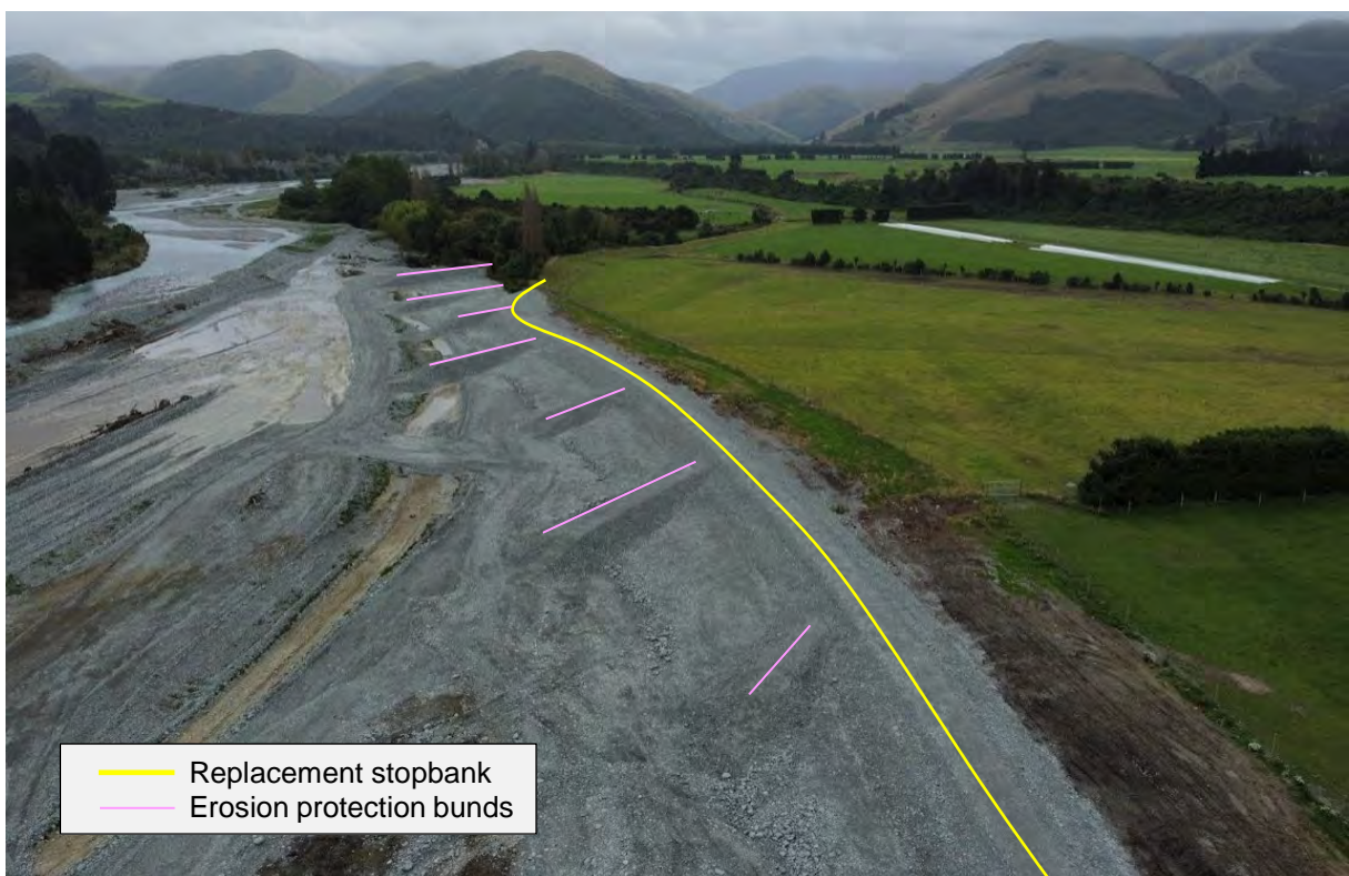
Figure 8-15: Orari at Inglis Rd Site B, Stopbank reinstated with erosion protection bunds. Topsoil to be added. 23/2/2022.
