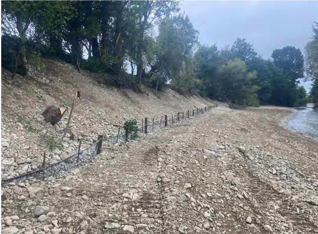
Figure 9-13: Waihi at SH79, Geraldine TLB downstream of bridge. Completed Heyman Fence repair. March 2022.
