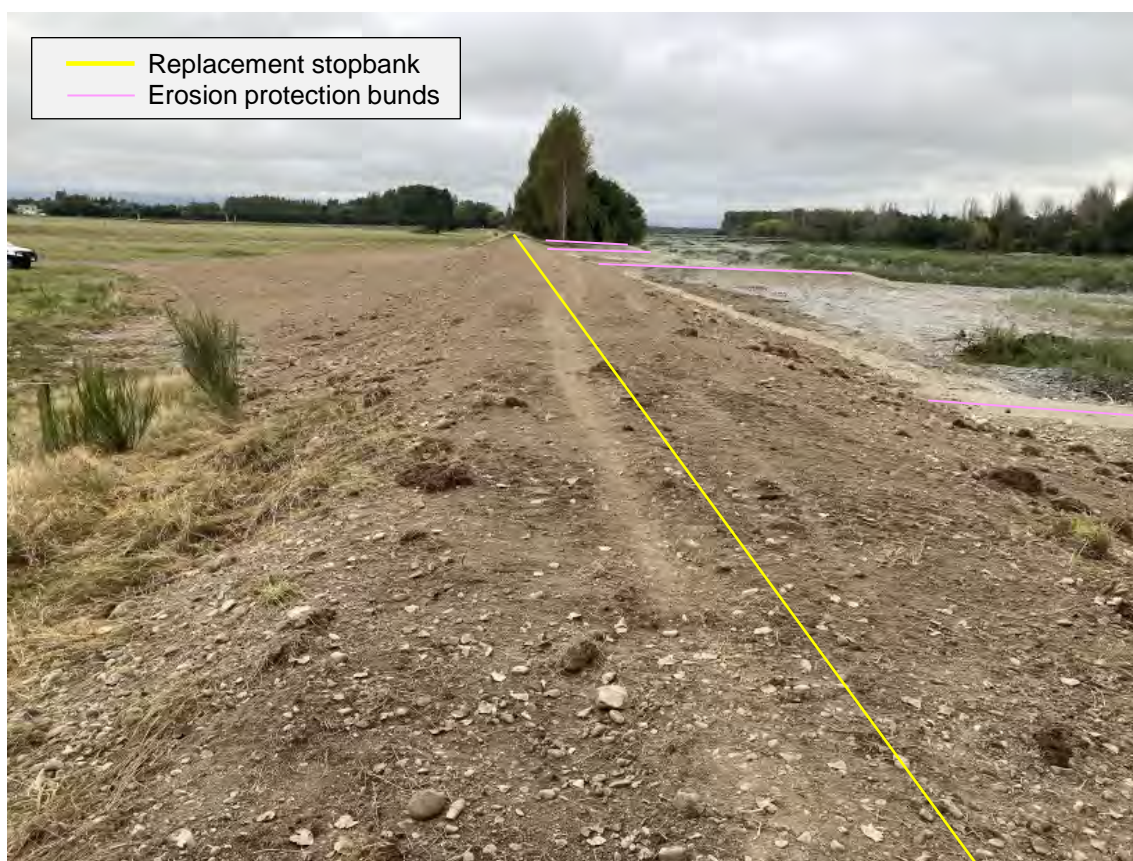
Figure 8-23: Orari at SH7 completed stopbank repairs. 18/3/2022.
