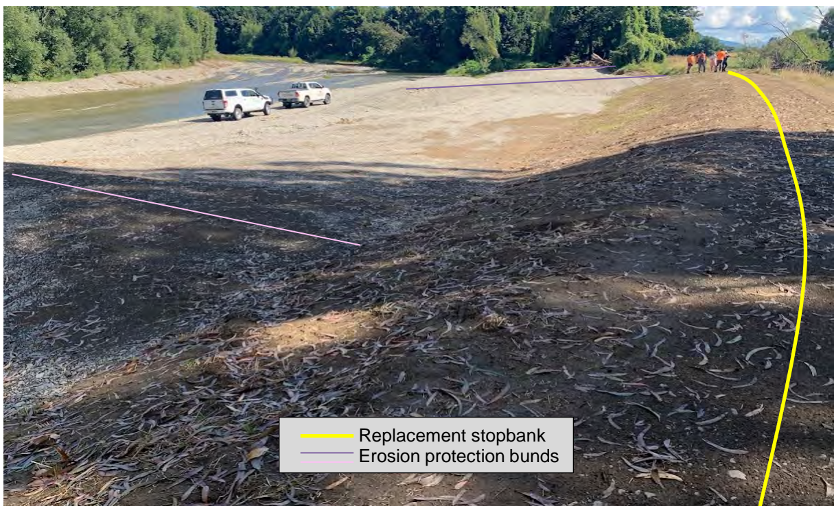
Figure 8-34: Waihi at Hawke Rd Site A, showing completed stopbank repairs and erosion protection bunds
