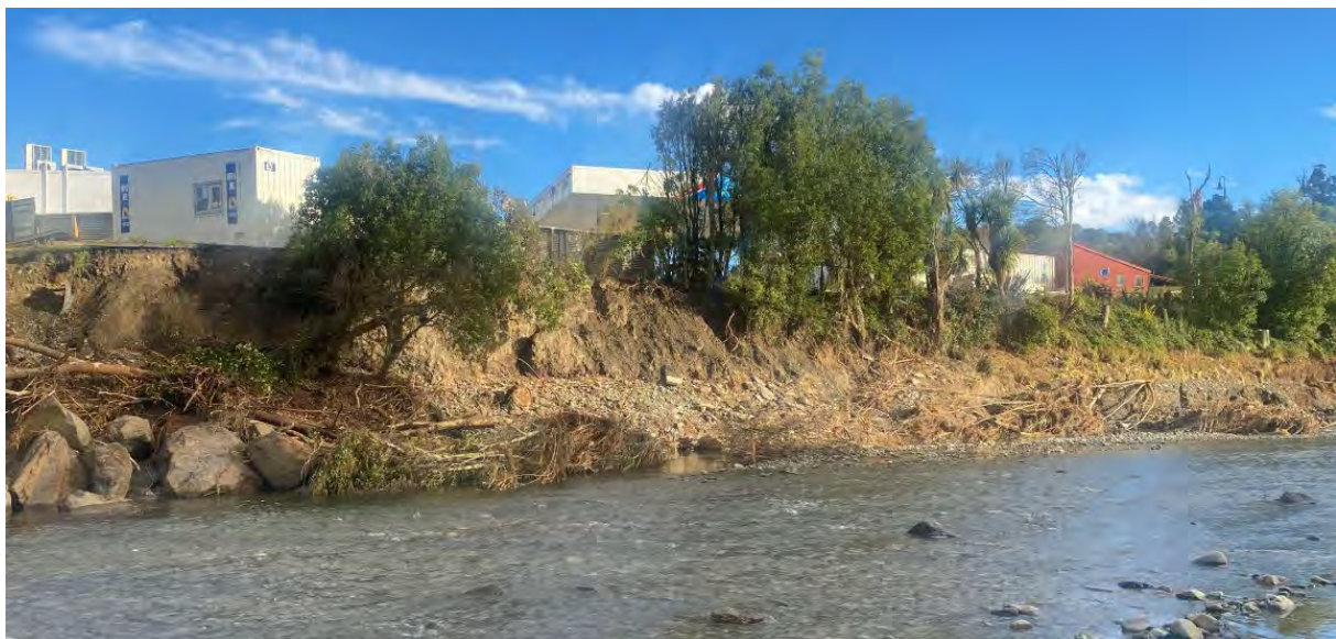
Figure 9-16: Waihi at Geraldine, NPD flood damage to rock groynes on TRB. June 2021.
