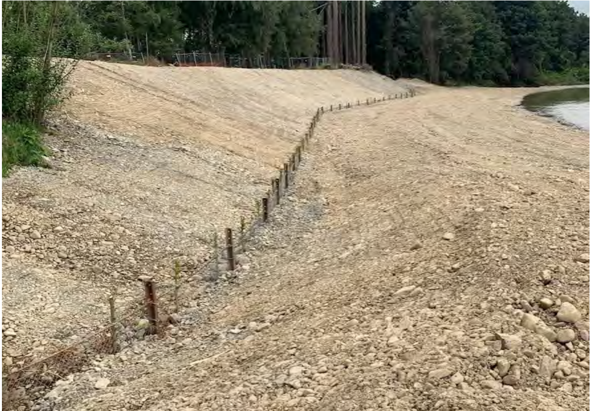
Figure 9-23: Waihi at Geraldine High School, completed Hayman Fence repair 23/2/2022.
