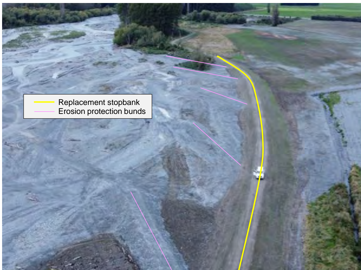
Figure 8-3: North Ashburton at Thompsons Track. Completed stopbank repair on 16 March 2022. Anchored tree protection and infill planting still to be done.
