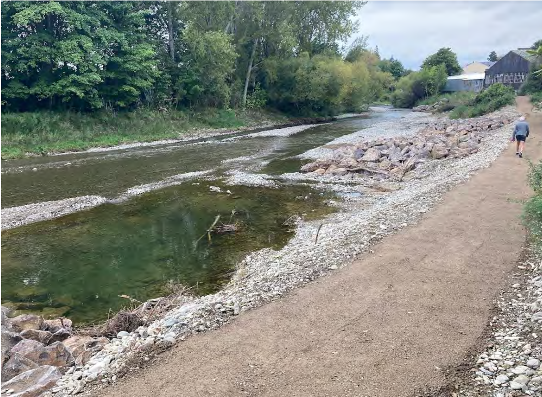
Figure 9-17: Waihi at Geraldine, NPD completed repair to rock groynes and access track on TRB. March 2022.
