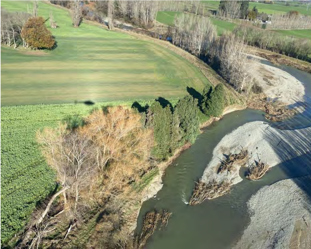
Figure 8-37: Waihi at Hawke Rd Site C looking downstream showing loss of stopbank and tree edge protection, June 2021.
