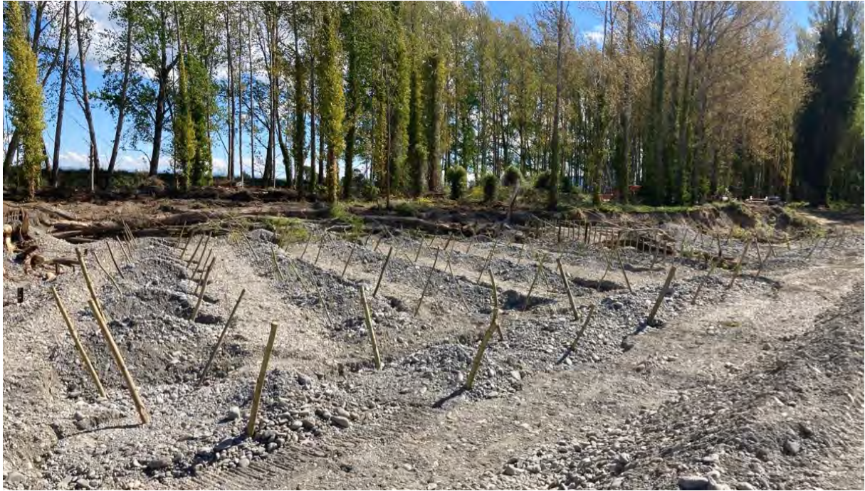
Figure 9-7: Orari at racecourse infill with willow poles.
