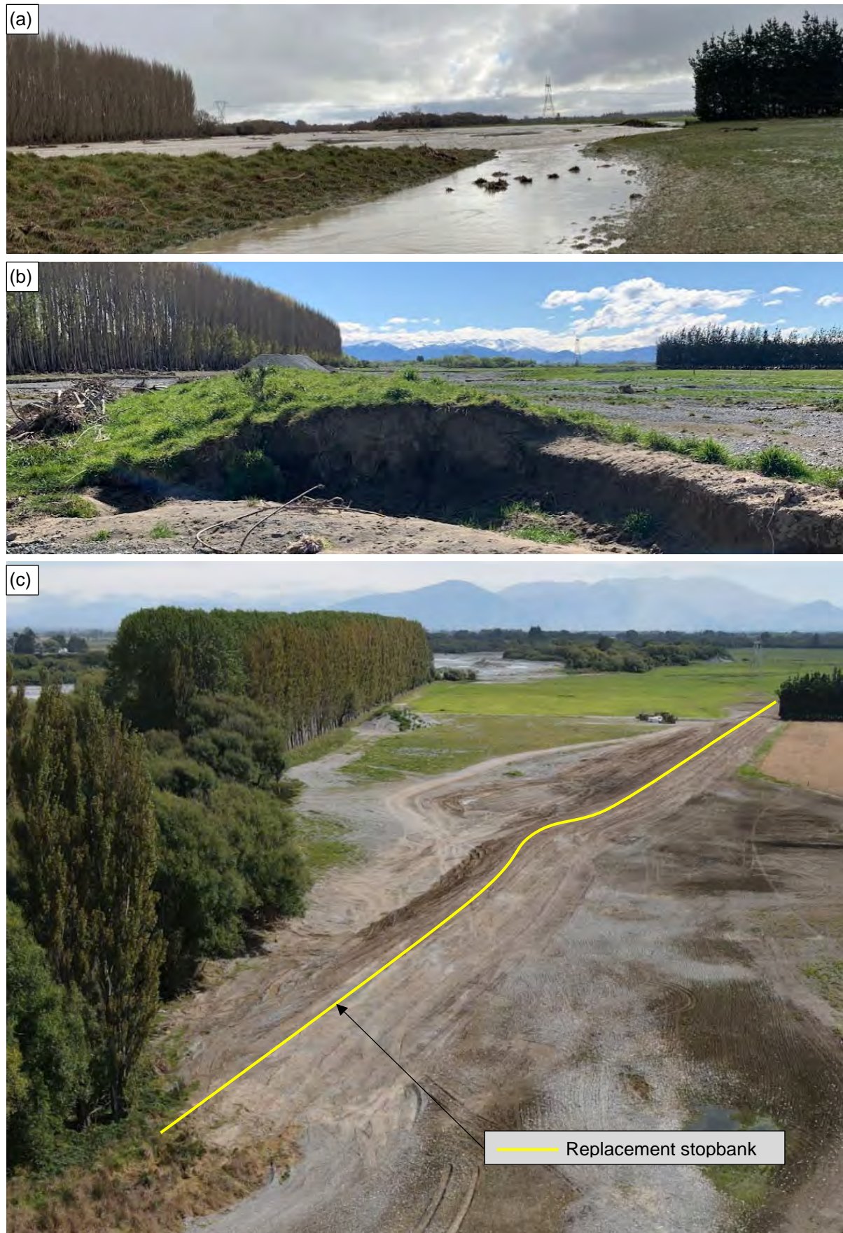
Figure 8-8: South Ashburton at Blacks Road looking upstream from lower end of remnant stopbank (a) early June 2021, (b) September 2021 and (c) on completion of replacement stopbank in February 2022.
