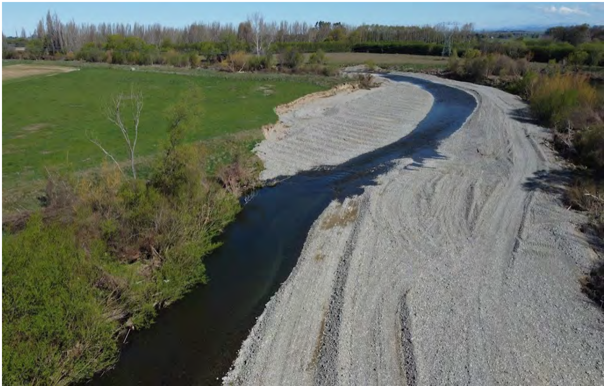
Figure 8-35: Waihi at Hawke Rd Site B looking downstream showing temporary bund work prior to permanent repairs, 28/9/2021.
