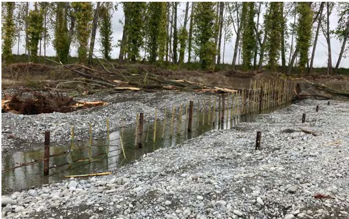
Figure 9-6: Orari at racecourse installation of rope and rail.
