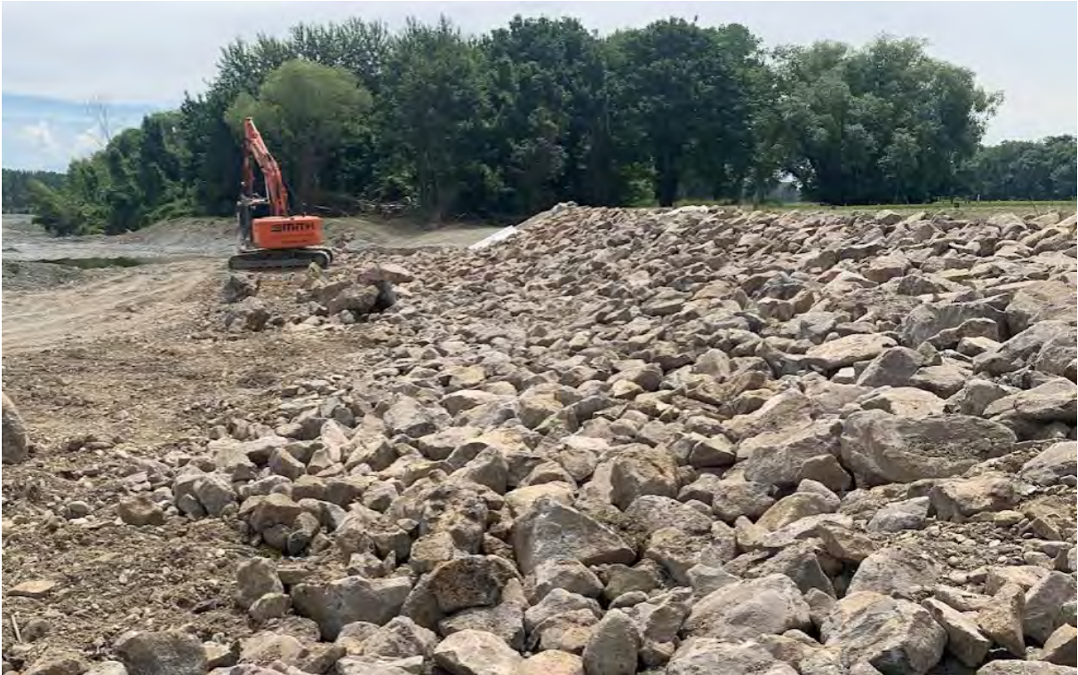
Figure 8-28: Orari at the railway bridge stopbank repair addition of rock riprap protection. November 2021.
