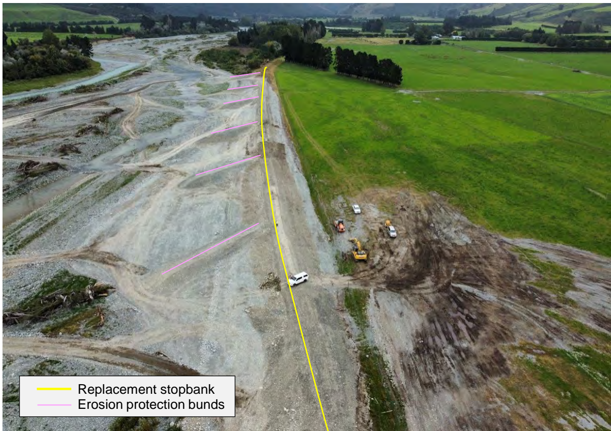
Figure 8-18: Orari at Inglis Rd Site C, looking upstream. Stopbank rebuild nearing completion, January 2022.
