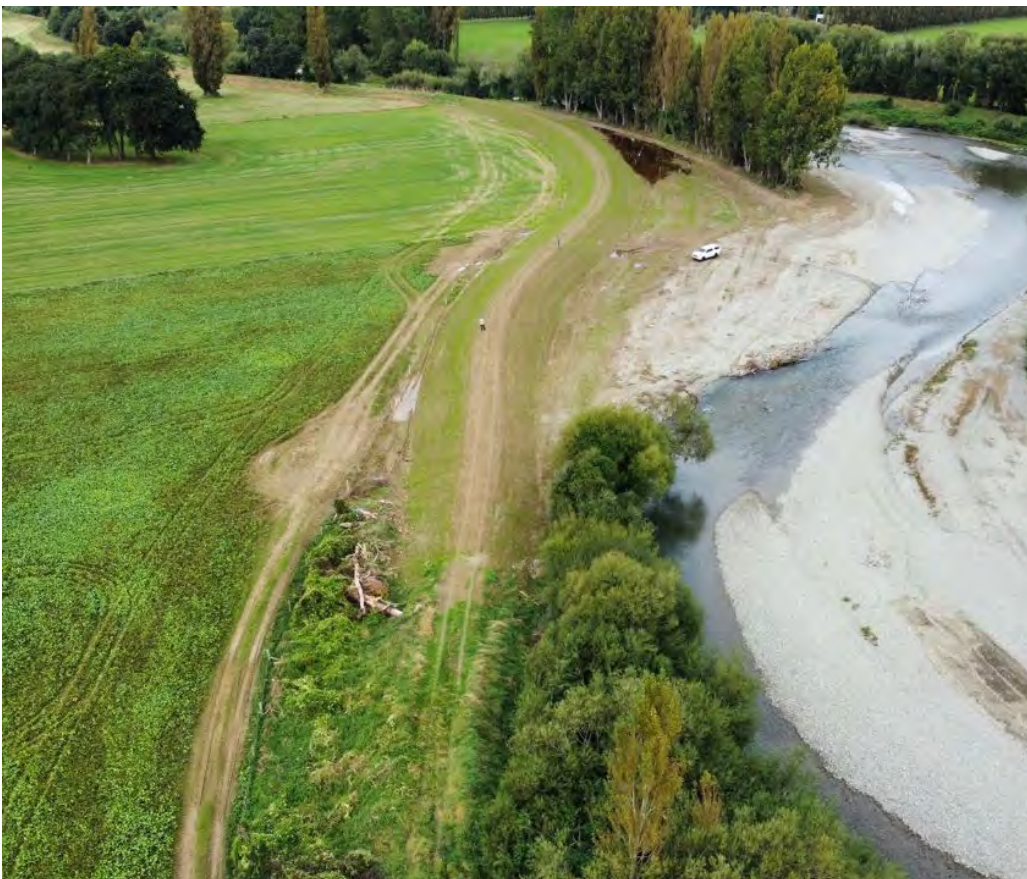
Figure 8-38: Waihi at Hawke Rd Site C looking downstream following completion of stopbank repairs, 23/2/2022.
