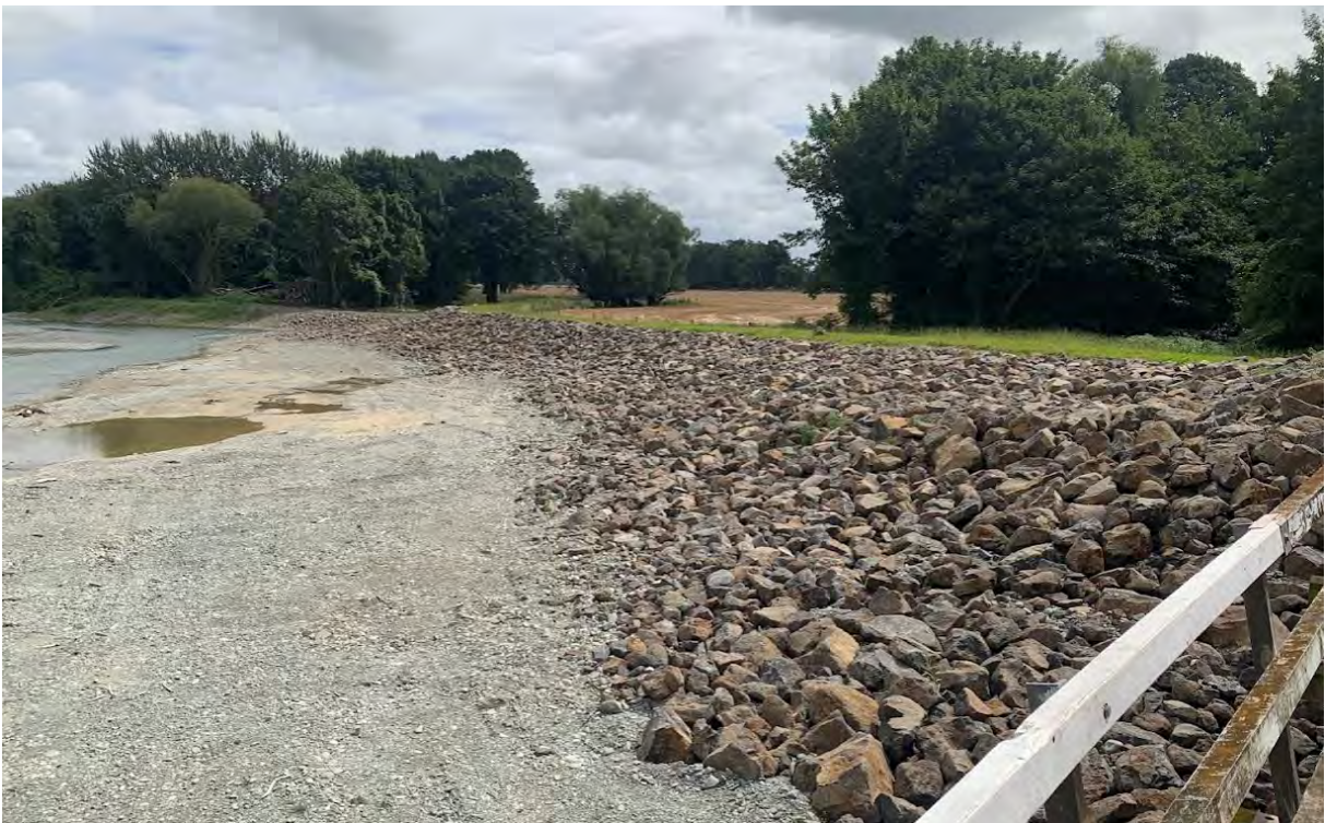
Figure 8-29: Orari at the railway bridge completed stopbank with rock protection. February 2022
