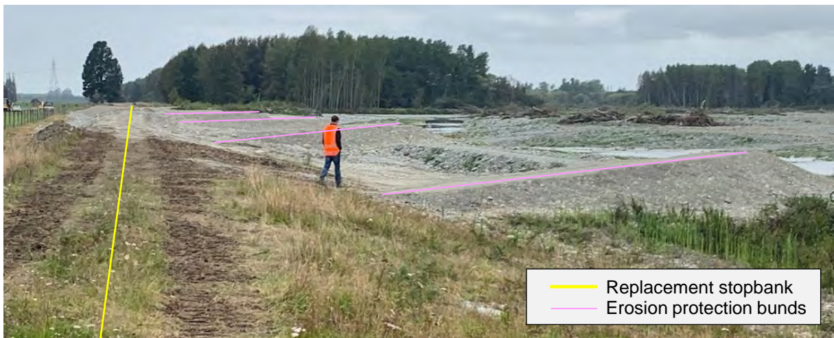
Figure 8-19: Orari at Inglis Rd Site C Stopbank completed to design height 7 of 9 erosion bunds complete, topsoil to follow, 23 February 2022.
