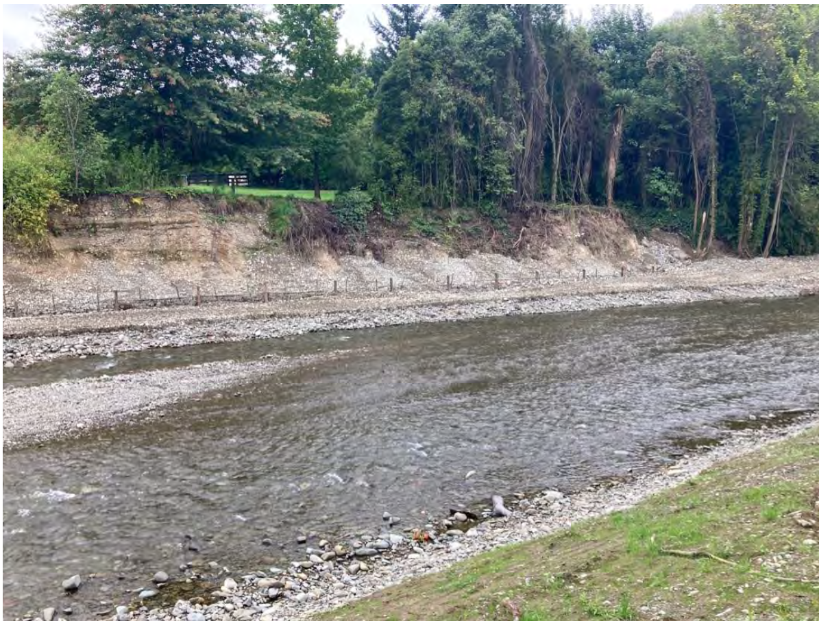
Figure 9-11: Waihi at SH79, Geraldine TRB upstream of bridge with completed Heyman Fence repair, March 2022.
