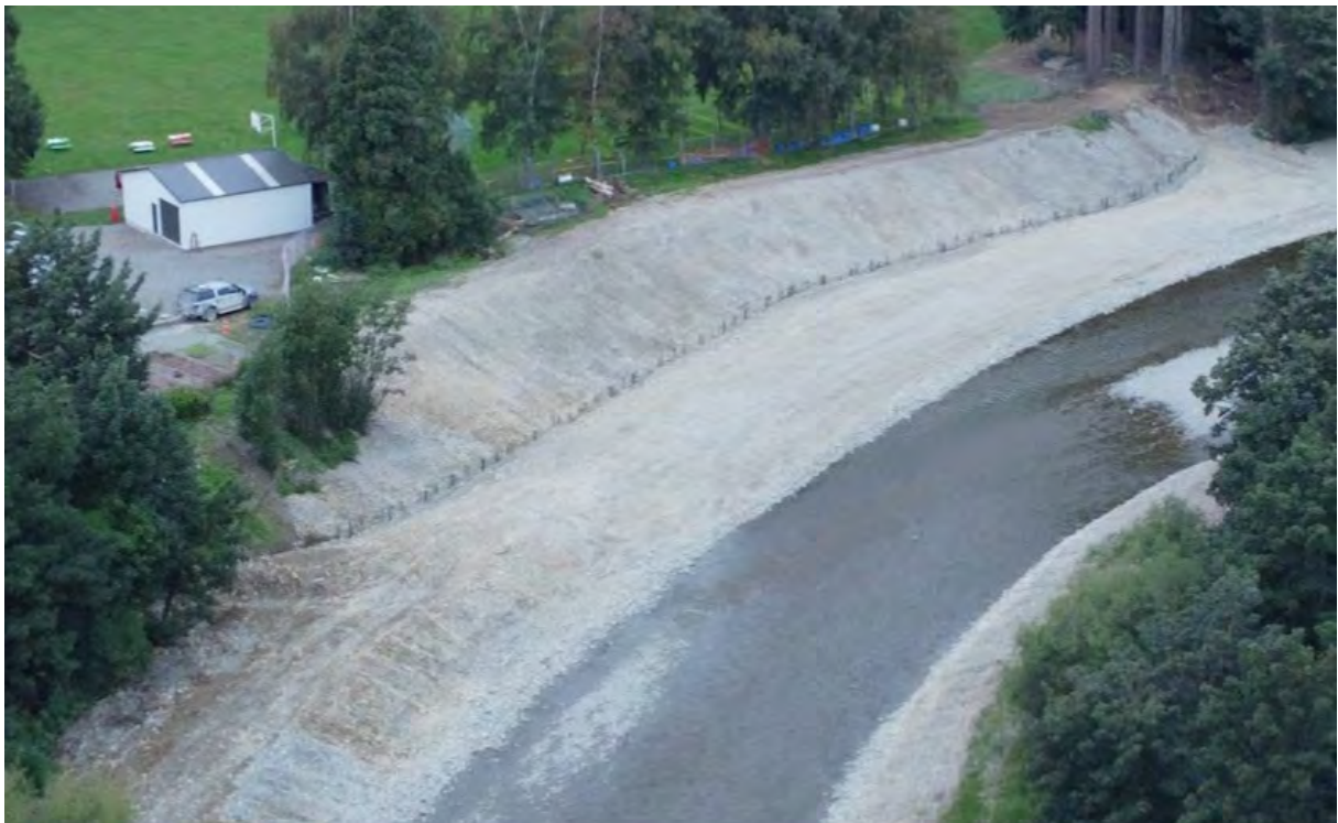
Figure 9-24: Waihi at Geraldine High School, completed Hayman Fence repair aerial view, March 2022.
