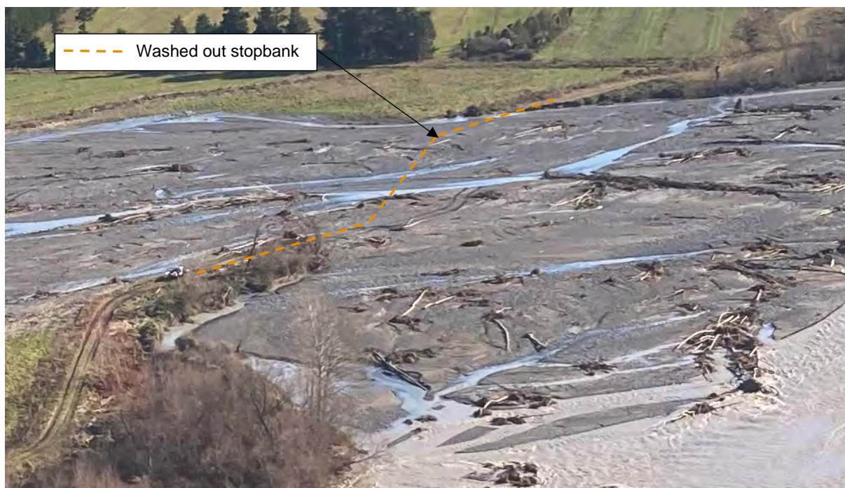
Figure 8-2: North Ashburton at Thompsons Track. Area of stopbank and tree edge protection loss on 3 June 2021.
