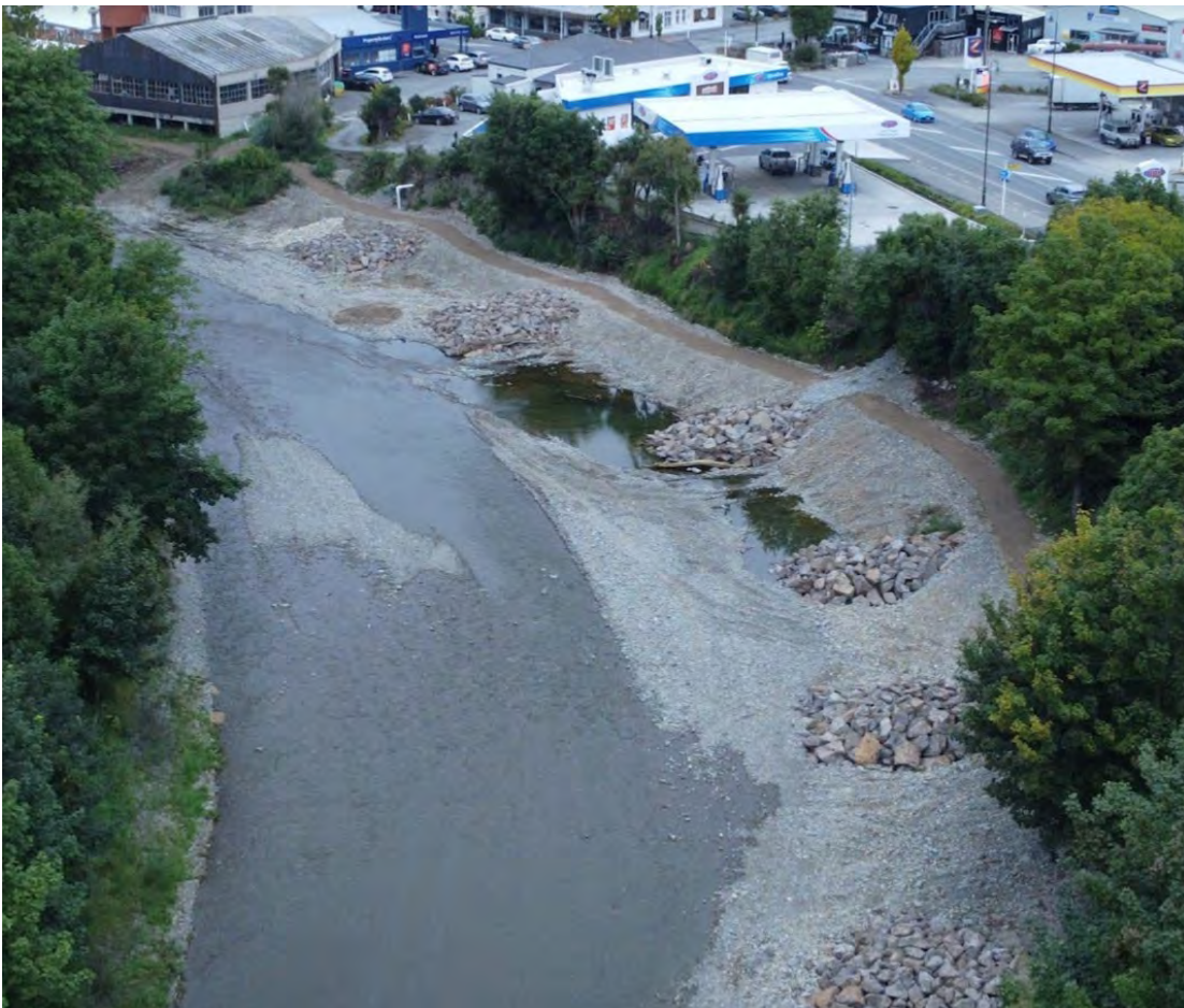
Figure 9-18: Waihi at Geraldine, NPD repaired rock groynes on TRB looking downstream. March 2022.
