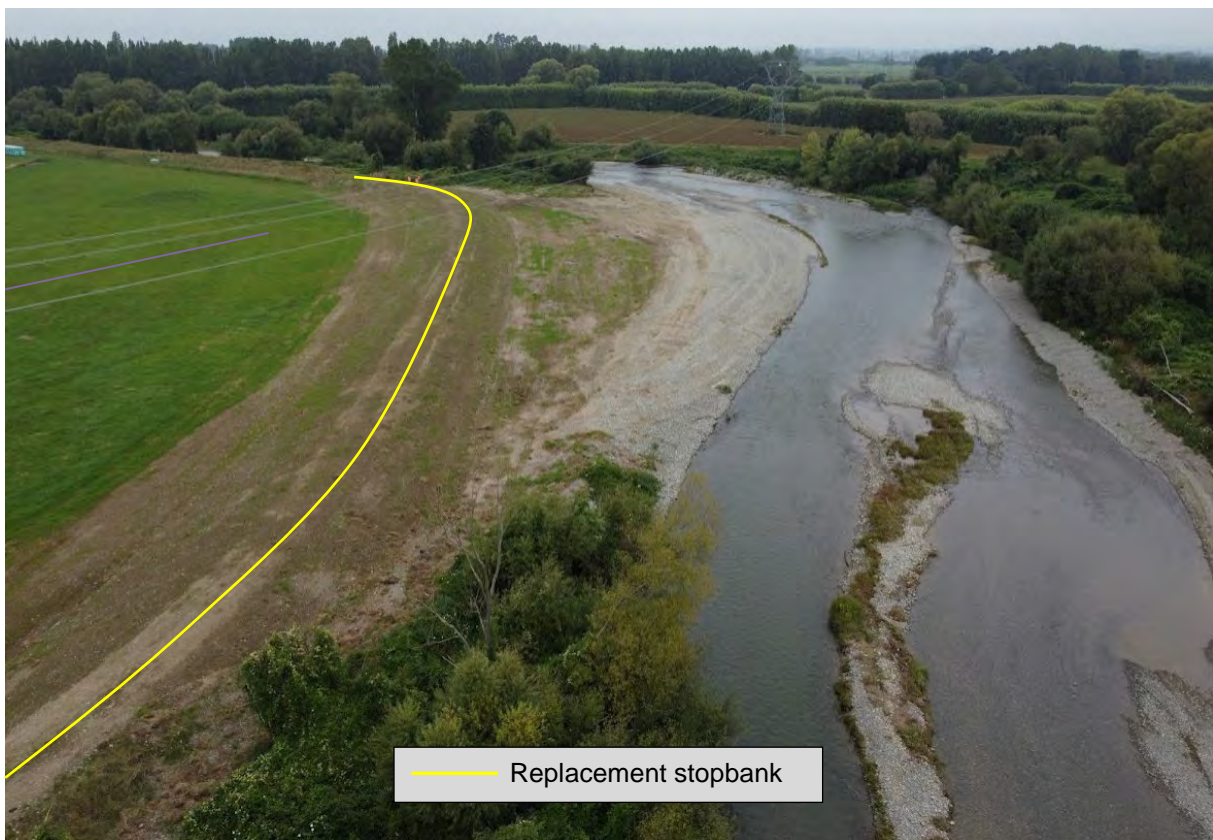
Figure 8-36: Waihi at Hawke Rd Site A, showing completed stopbank repairs and erosion protection bunds, 9/2/2022.
