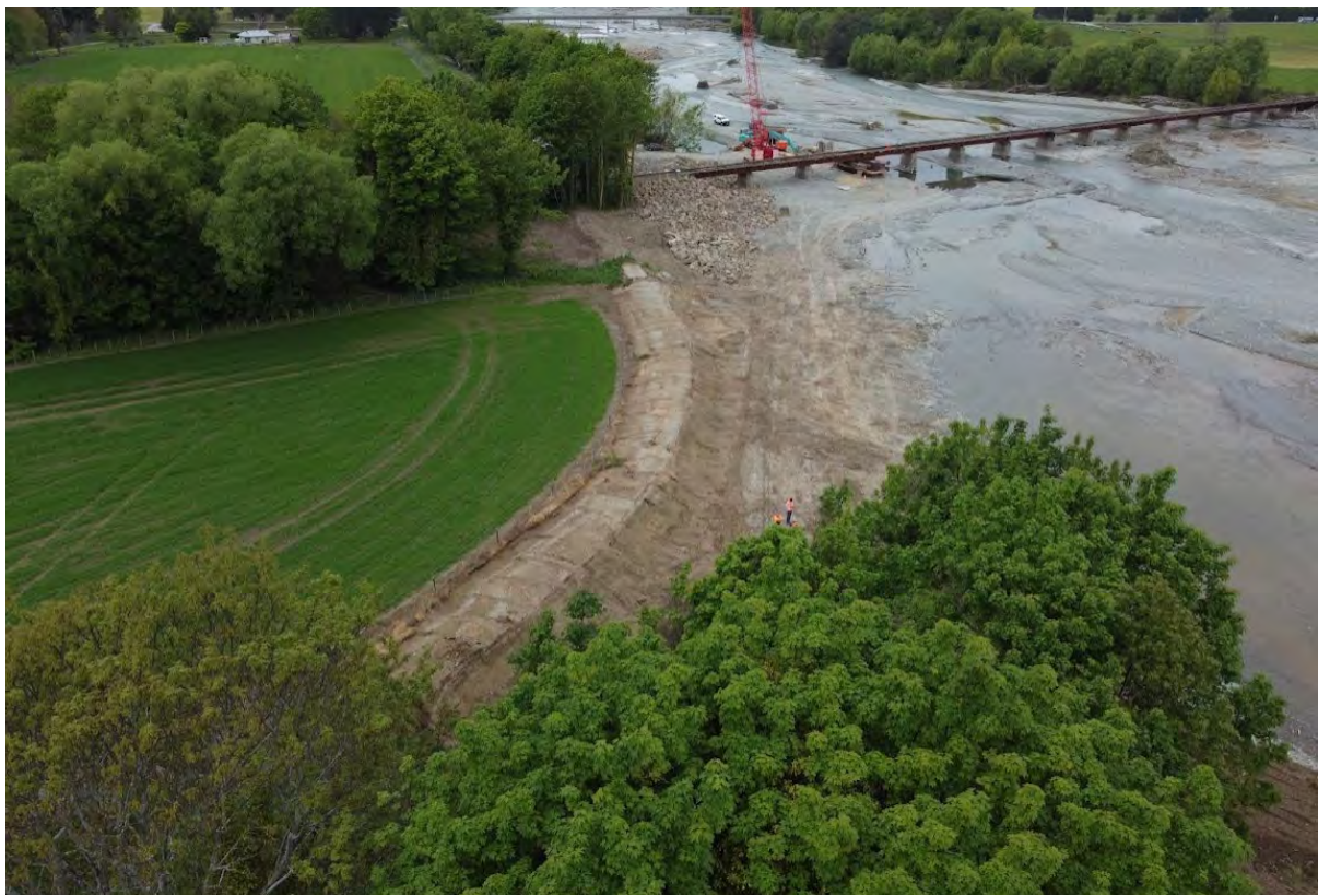
Figure 8-27: Orari at the railway bridge stopbank repair prior to adding or riprap rock protection. October 2021.
