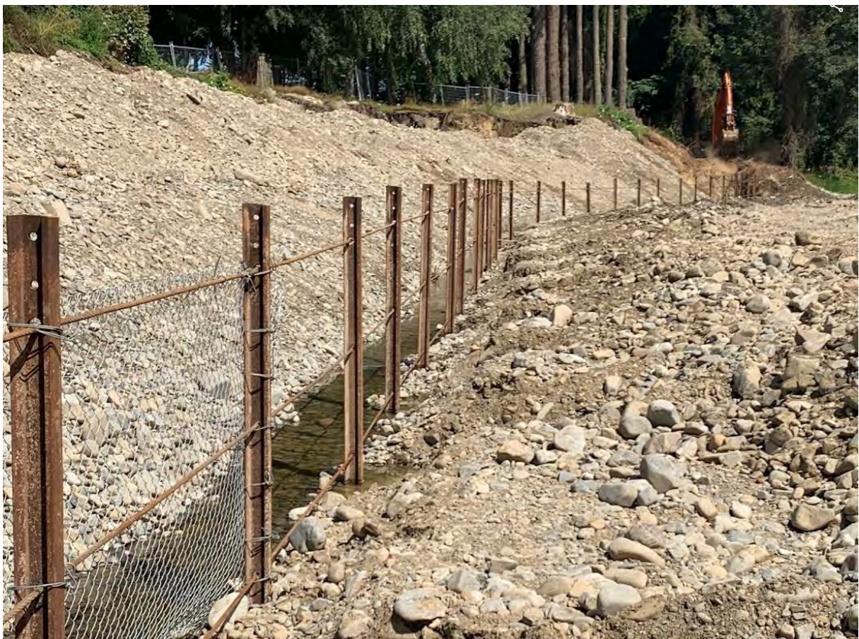
Figure 9-22: Waihi at Geraldine High School Hayman Fence being implemented 27/1/2022.
