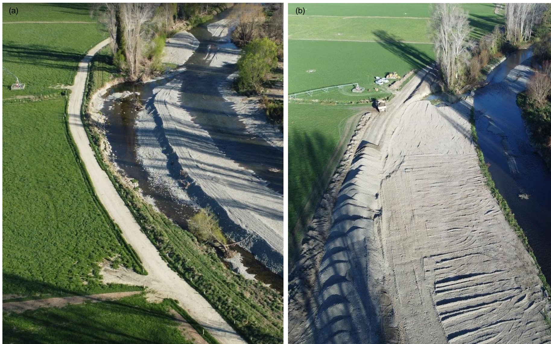
Figure A-3: Aerial of Waihi at Beeby Rd (a) after temporary repairs and (b) during stopbank reinstatement.
