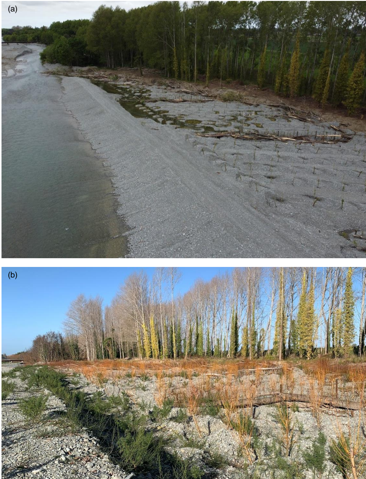
Figure A-5: Orari at racecourse (a) after completion of rope and rail lines (October 2021) and (b) showing growth of poles by June 2022.
