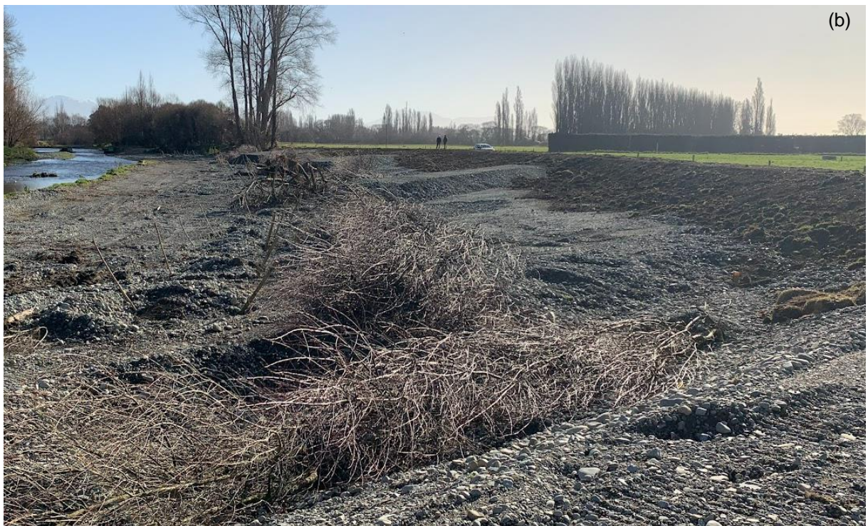
Figure A-2: Waihi at Beeby Rd (a) before repair, (b) after stopbank reinstatement and installation of anchored tree protection.
