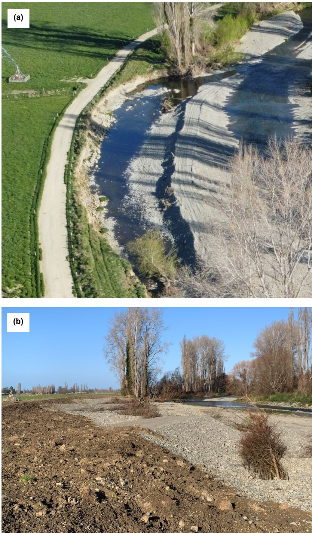
Figure A-5: Waihi River at Beeby Rd, (a) after 2021 flood with temporary bund, and (b) following completion of stopbank repair, erosion protection bunds and ATP (6 July 2022).
