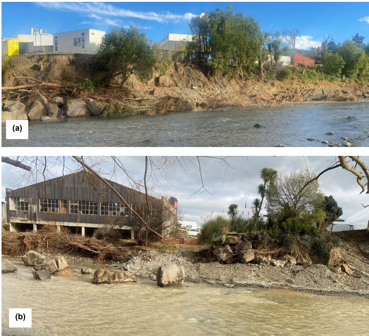
Figure A-8: Waihi at Geraldine NPD following 2021 flood showing (a) bank scour and (b) displacement of rock groyne.
