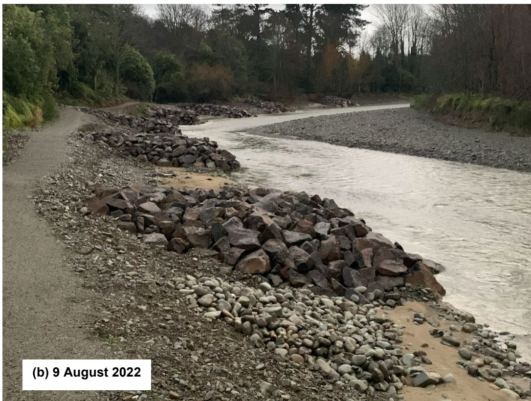
Figure A-9: Waihi at Geraldine NPD showing rock groyne repair (a) after completion and (b) after high July/August high flows (9 August 2022).
