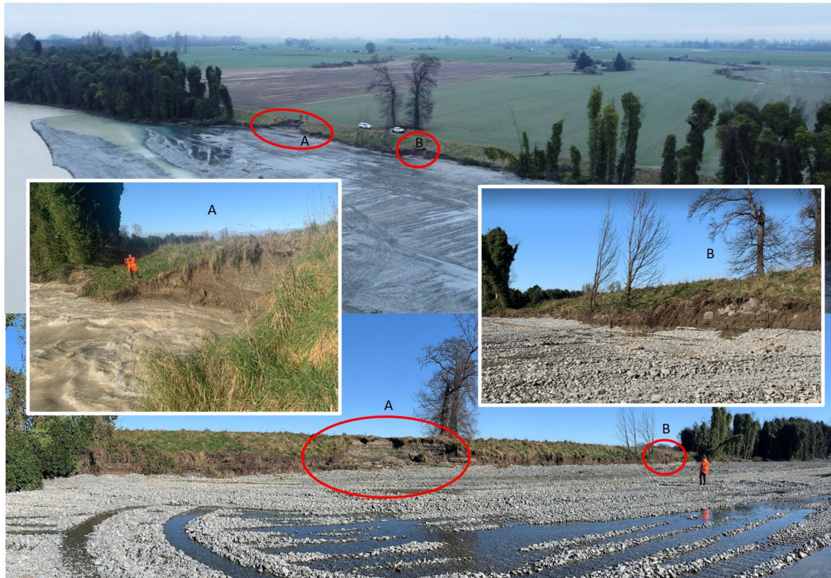
Figure B-9: Orari at Stewart Road, stopbank damage at A and B and scour of 230m length of stopbank berm.
