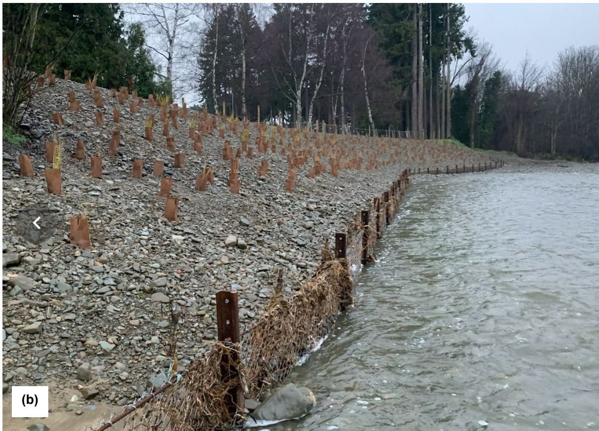
Figure A-7: Waihi at Geraldine High School (a) following flood damage before repair, (b) after repair of embankment with Heyman Fence and native planting on bank holding up well in 2022 high flows (9 August 2022).
