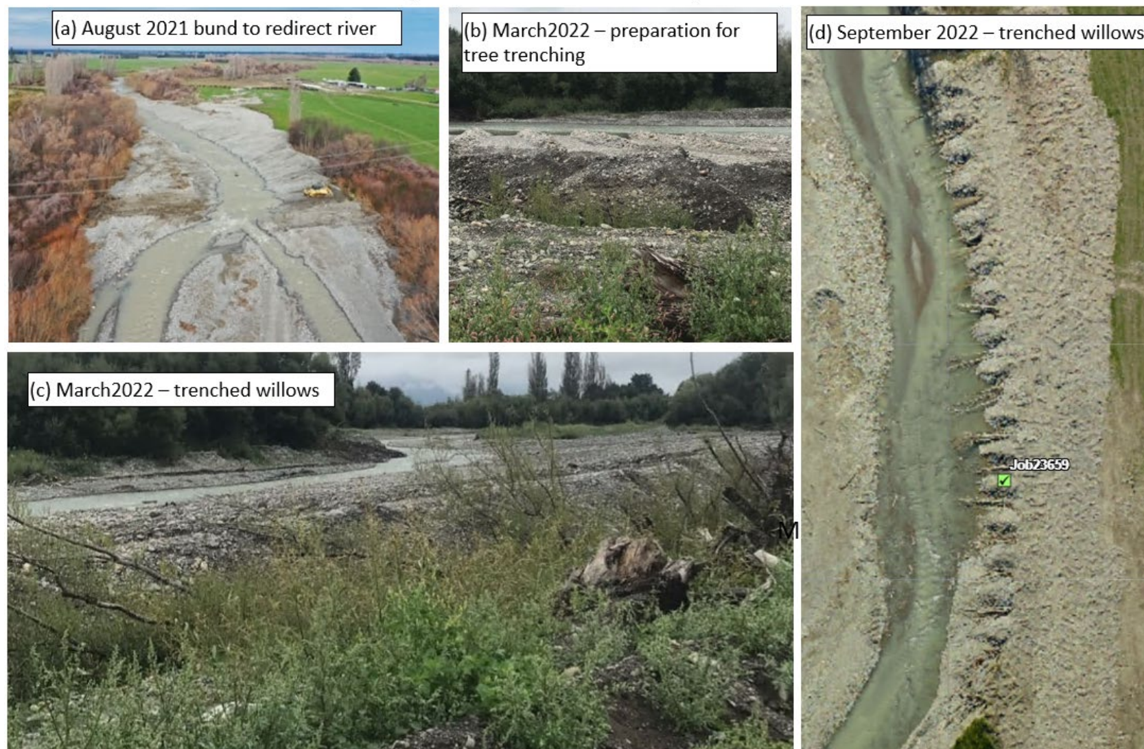
Figure A-15: Taylors Stream repair details (a) in August 2021, (b) and (c) trenched willows in March 2022, and (d) more substantial trenched willows, September 2022.
