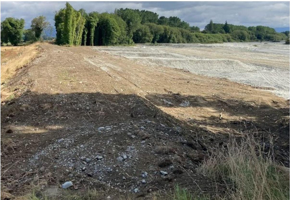
Figure A-1: Orari at Stewart Road (a) tree edge protection loss and stopbank scour, (b) repaired stopbank, berm and erosion protection bunds, awaiting ATP and infill planting.
