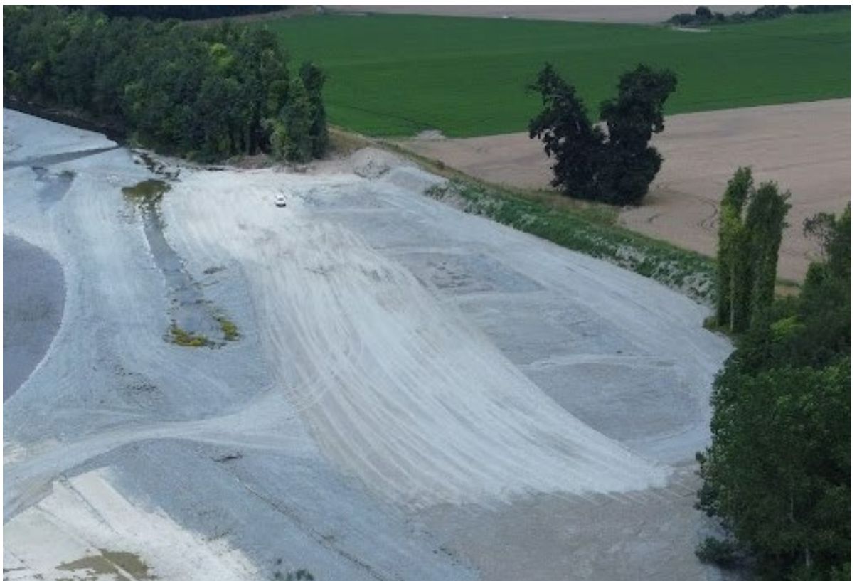
Figure A-2: Orari at Stewart Road aerials of (a) flood damage, (b) repaired stopbank, berm and erosion protection bunds, awaiting ATP and infill planting.
