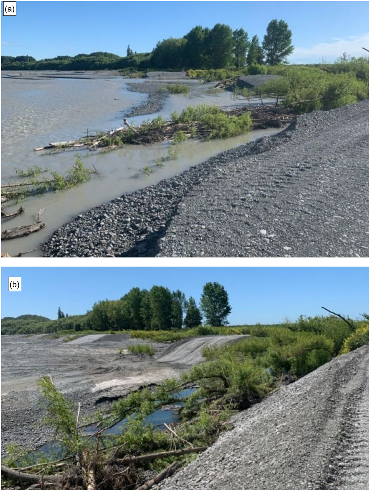
Figure A-1213: Ashburton main stem at River Road, (a) following winter 2022 damage-on-damage, and (b) after minor repairs undertaken in November 2022.
