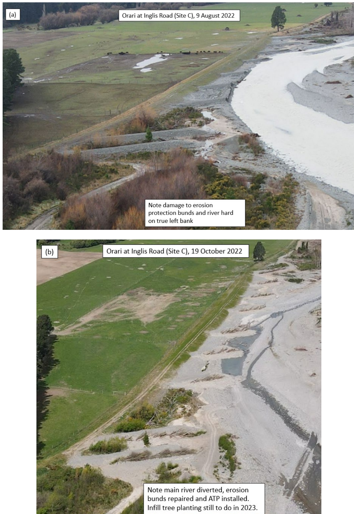
Figure A-7: Orari at Inglis Road, Site C: (a) damage to erosion protection bunds July/Aug 2022, (b) erosion bunds repaired and ATP complete, October 2022.
