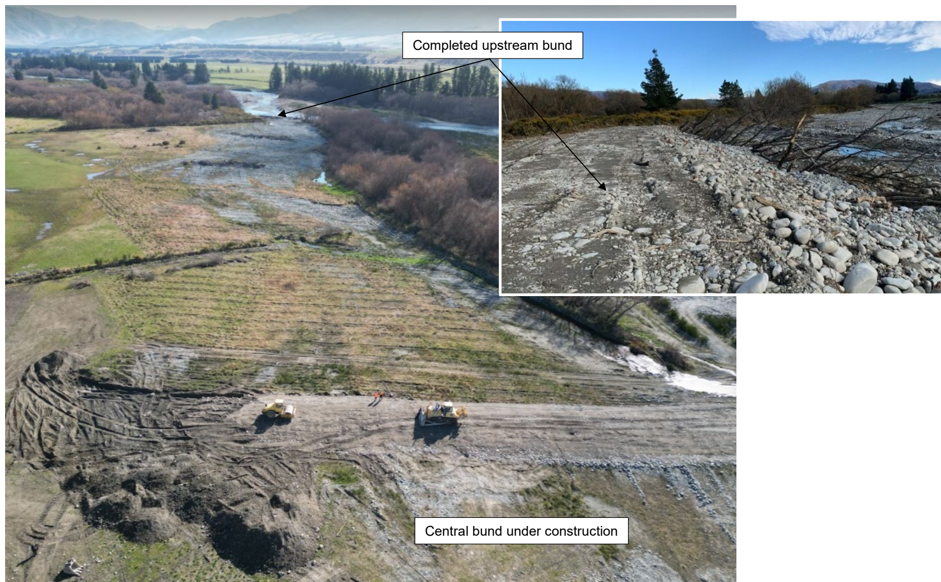
Figure B-10: Ashburton South at Mount Somers, central bund under construction (22 Aug 2023), with completed upstream bund with ATP (inset), early October 2023.
