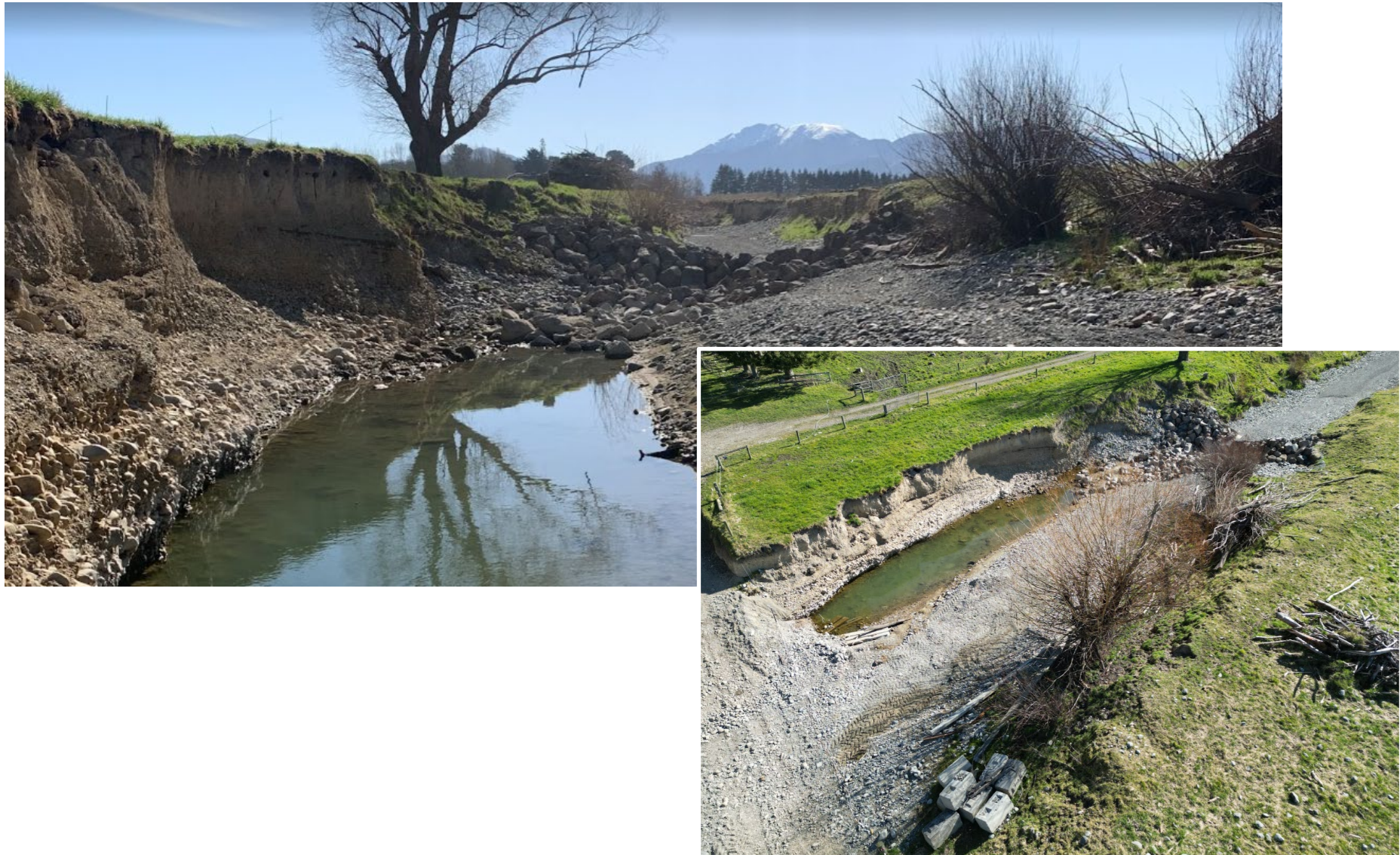
Figure C-11: Sweetwater Creek, weir 6 requiring mitigation following damage-on-damage due to winter 2023 high flows.
