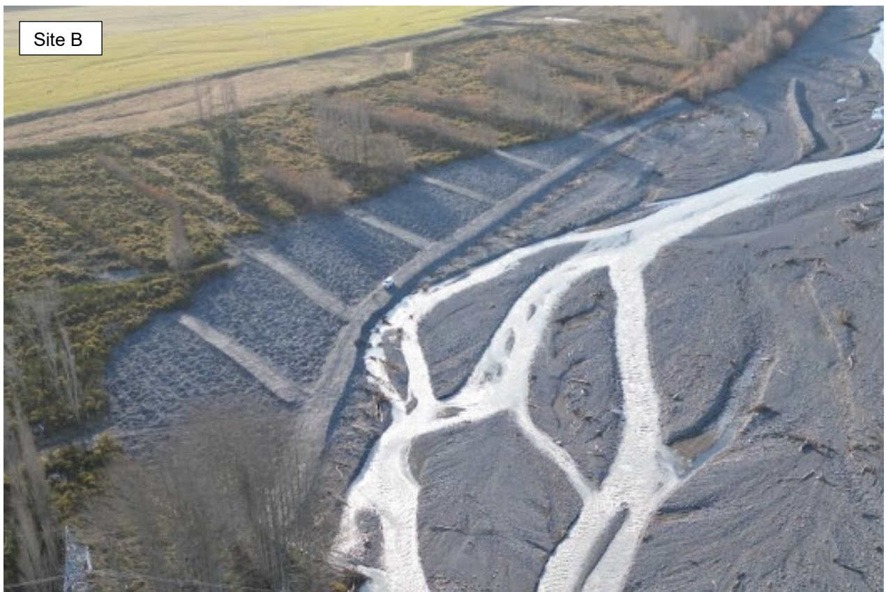
Figure B-7: Ashburton North at RDR, completed repairs at Site B, showing minor damage following July 2023 high flows (photos 23 August 2023).
