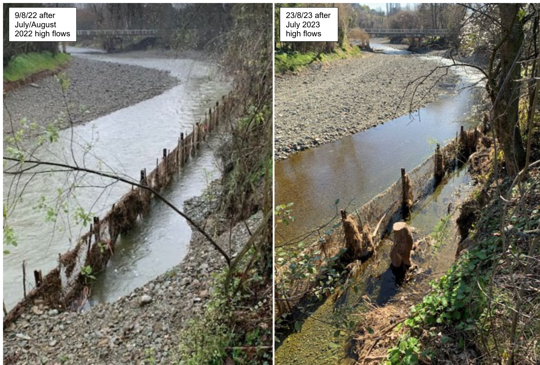
Figure C-9: Waihi at Geraldine, Heyman fence downstream of SH79 showing damage-on-damage due to winter high flows in 2022 and 2023.
