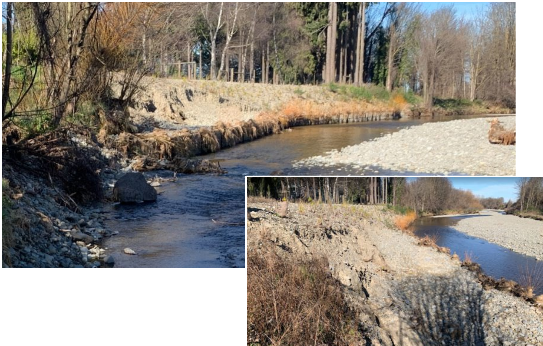
Figure C-10: Waihi at Geraldine High School, Heyman fence at showing damage-on-damage due to winter 2023 high flows.
