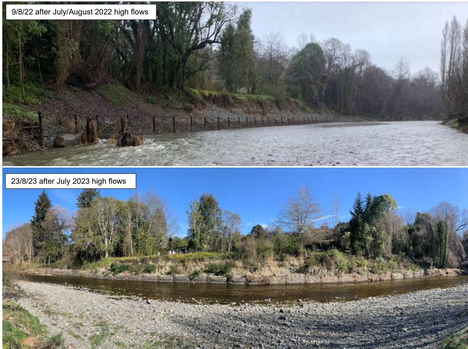
Figure C-8: Waihi at Geraldine upstream of SH79 showing damage-on-damage scour due to winter high flows in 2022 and 2023.
