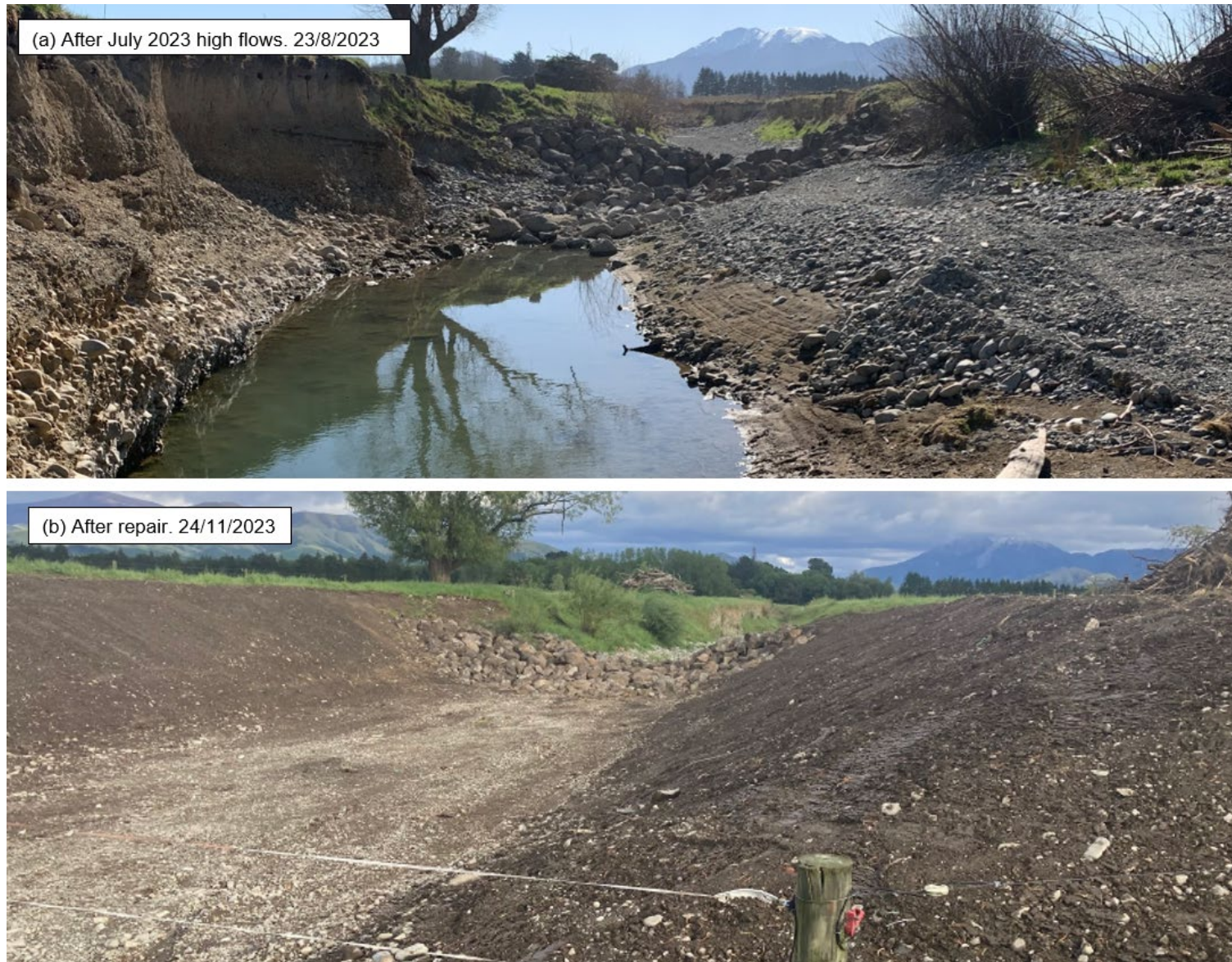
Figure A-4: Sweetwater Creek rock weir, (a) following 2023 high flow, and (b) after repair.
