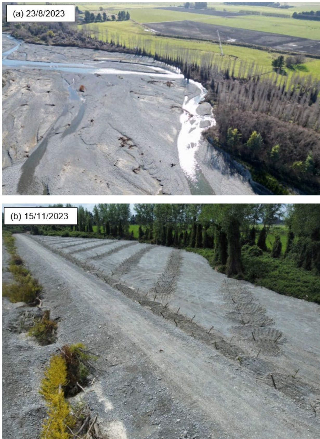
Figure A-7: Orari River at Taylors Road TLB (a) following flood damage in 2021 exacerbated in 2022 and 2023 and (b) after repair in 2023.
