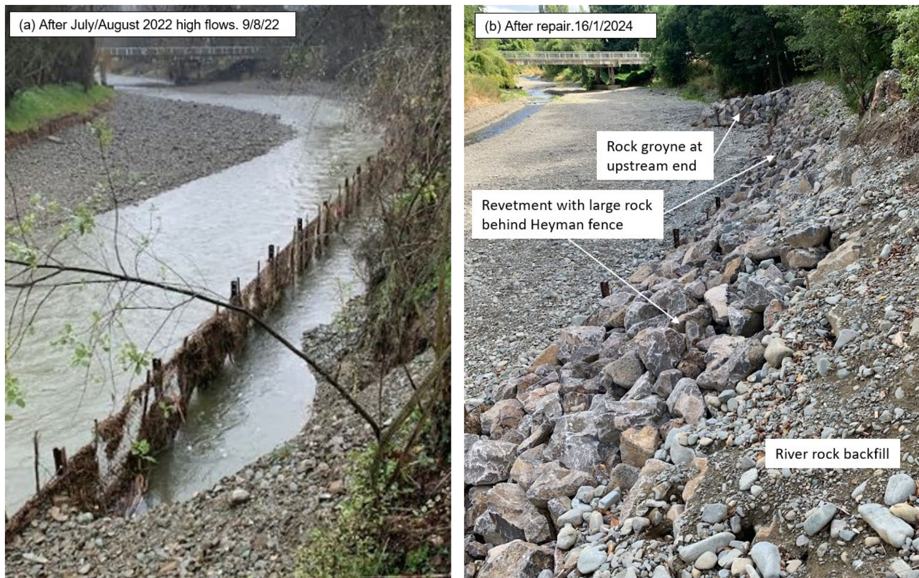
Figure A-2: Waihi at Geraldine, Heyman fence on left bank downstream of SH79, (a) before and (b) after repair.
