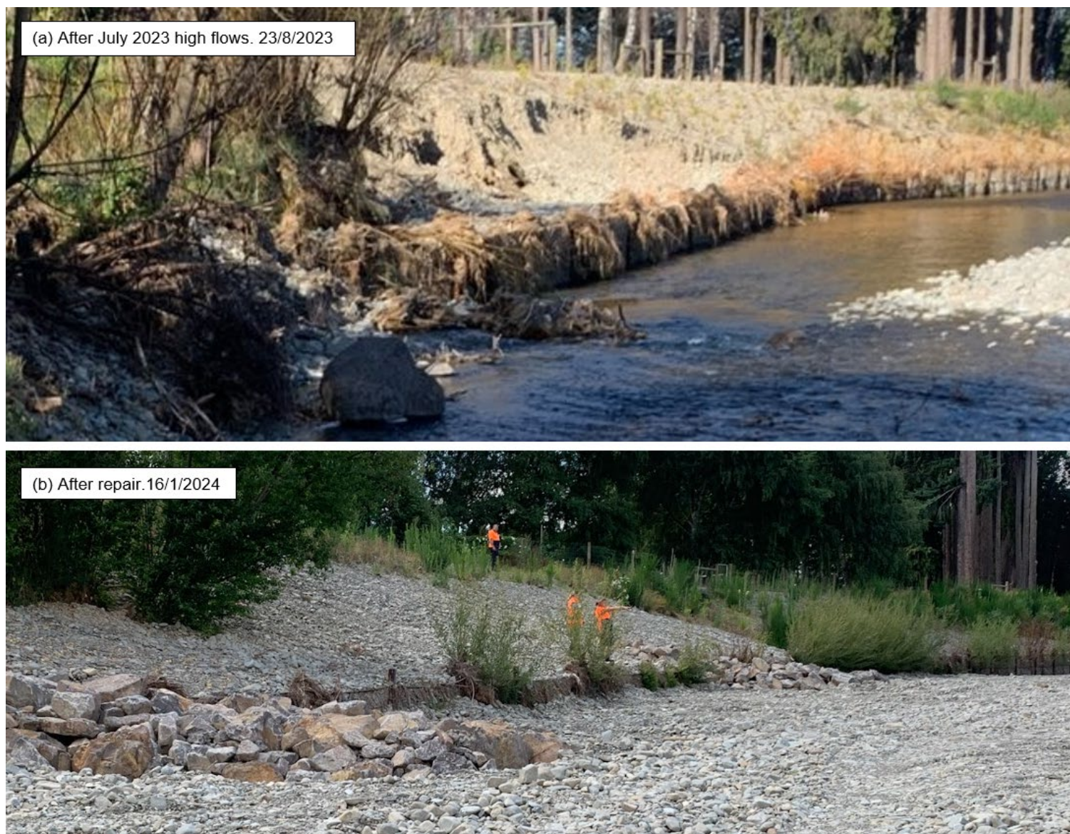
Figure A-3: Waihi River at Geraldine, Heyman fence on left bank at Geraldine High School, (a) before and (b) after repair.
