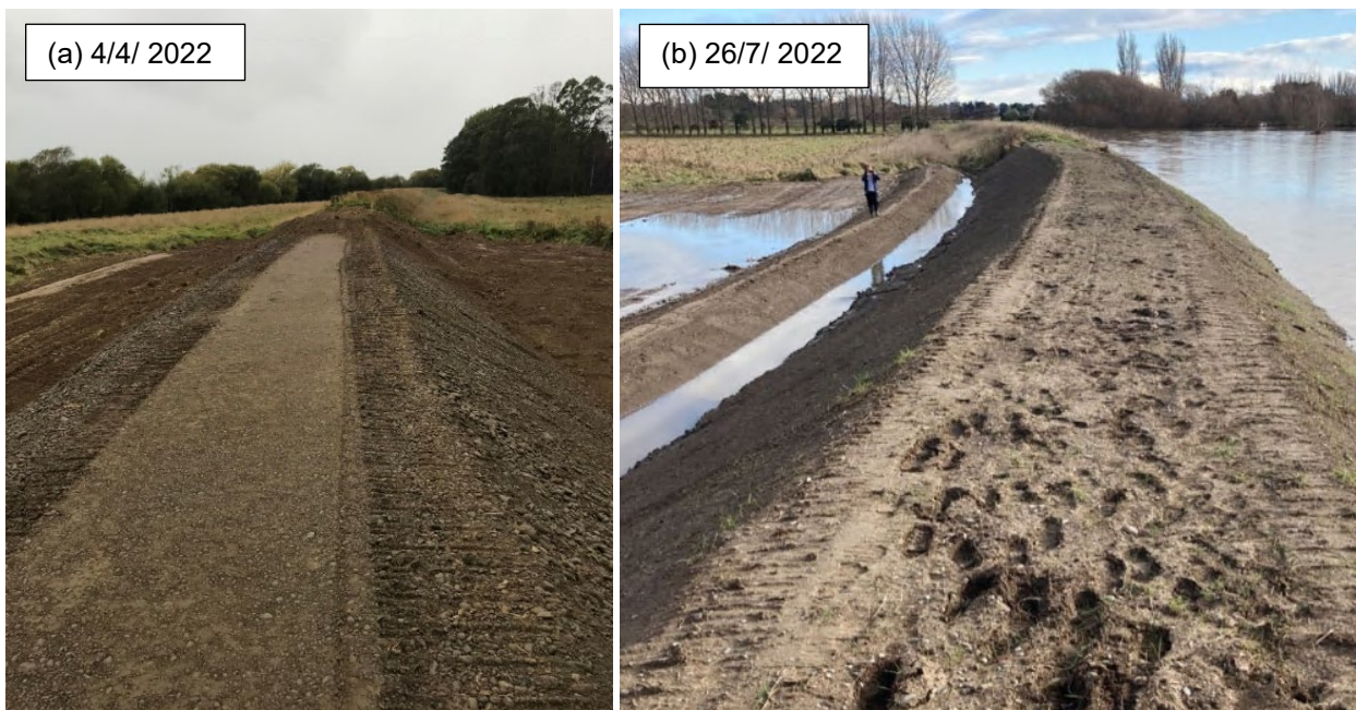
Figure A-9: Selwyn River stopbank following initial stopbank repair (a) April and (b) July 2022.
