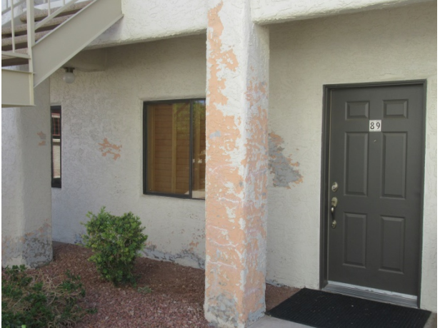
Stucco façade, note – building previously being painted
