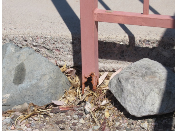
Corroded post at sidewalk across from Buildings 4 and 5
