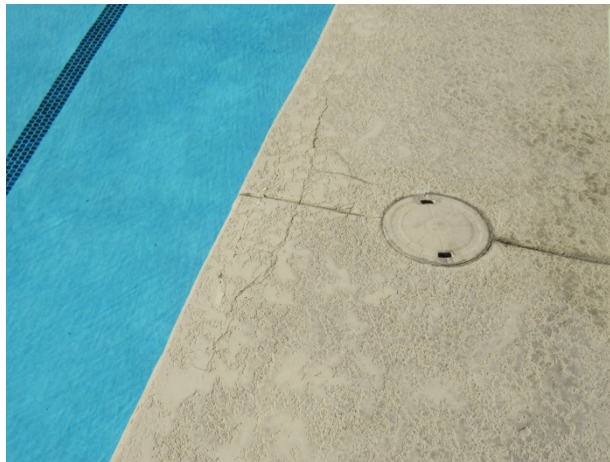
Cracks near edge
