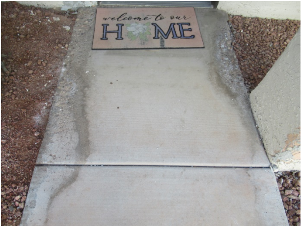
Spalled concrete
