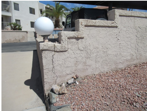
Light fixture, note perimeter wall crack
