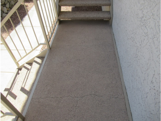
Cracks at concrete landing
