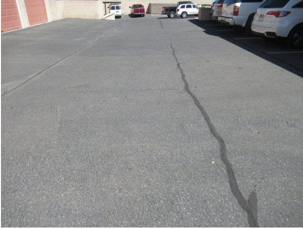
Asphalt pavement overview
