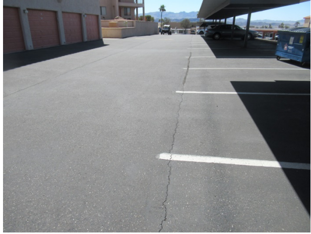
Asphalt pavement overview
