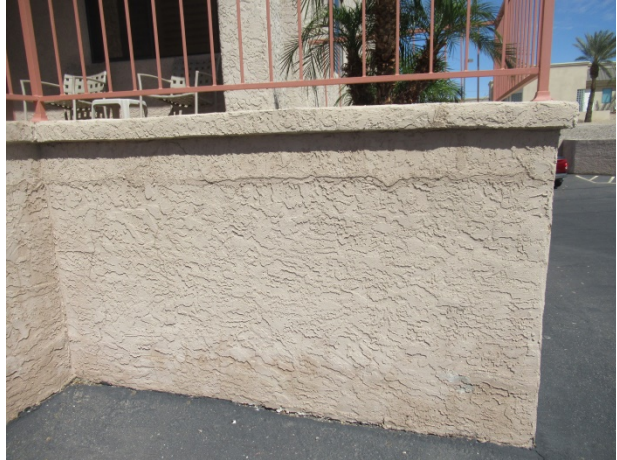
Stucco cracks
