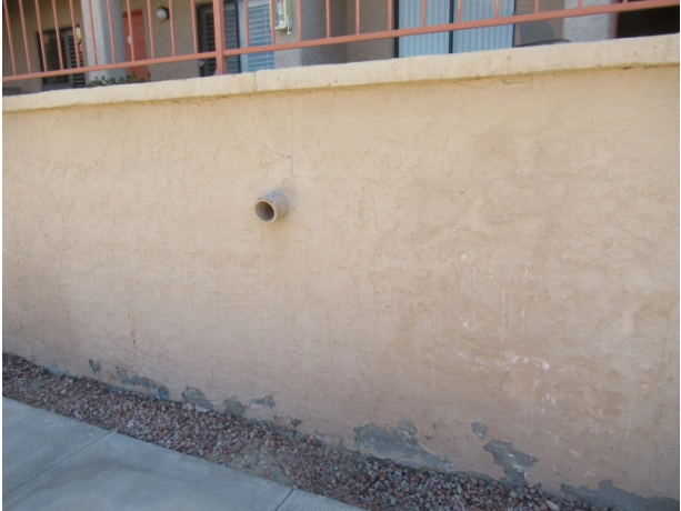
Coating deterioration
