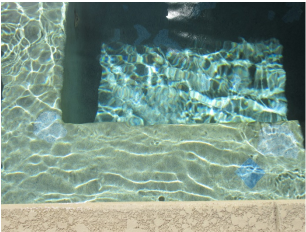
Chipped plaster at spa #1
