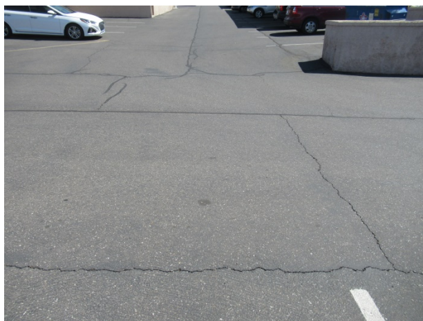
Various cracks near southwest entrance
