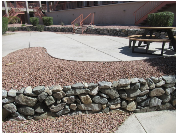
Stone retaining walls
