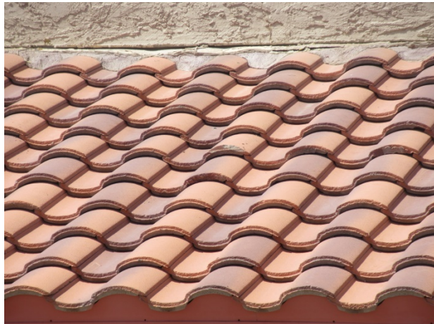
Minor chipped tile
