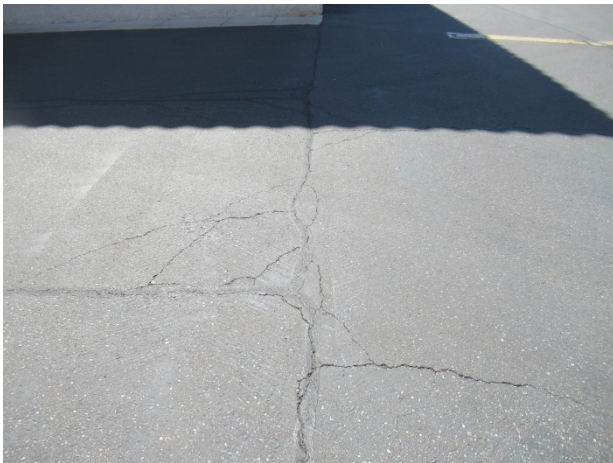
Pavement cracks
