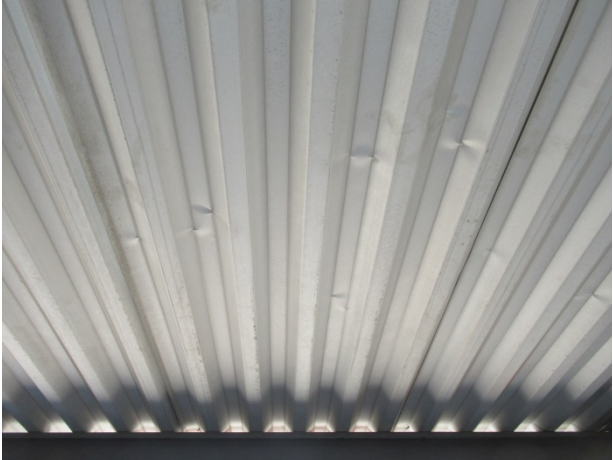
Dented roofing
