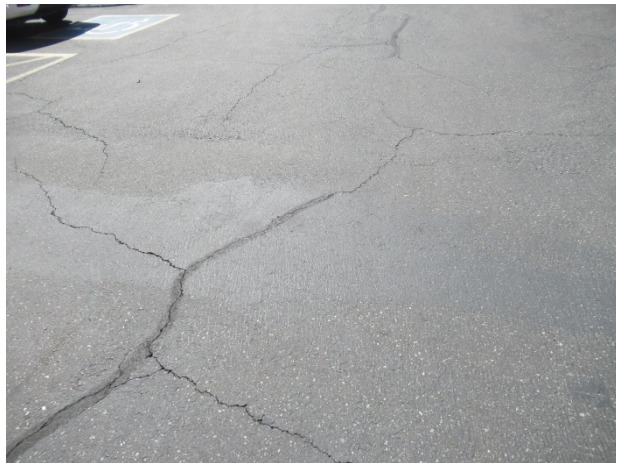
Pavement cracks
