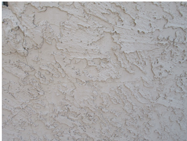
Stucco cracks
