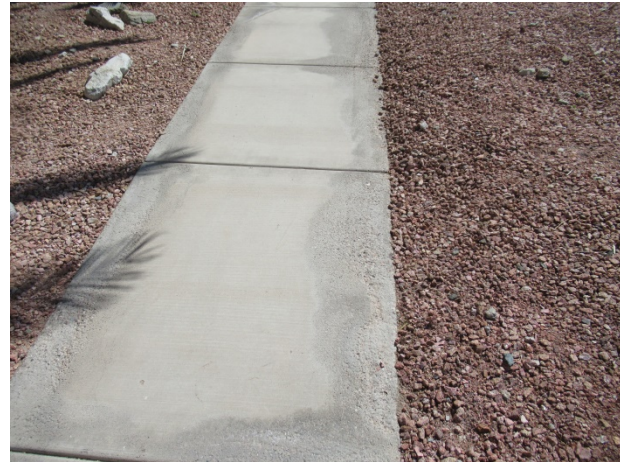
Spalled concrete
