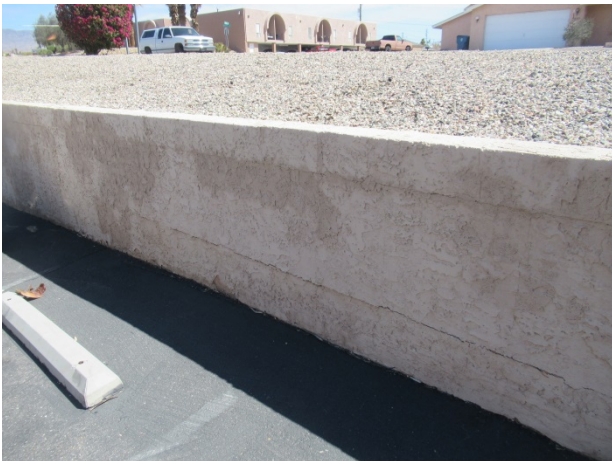
Deterioration at perimeter retaining wall
