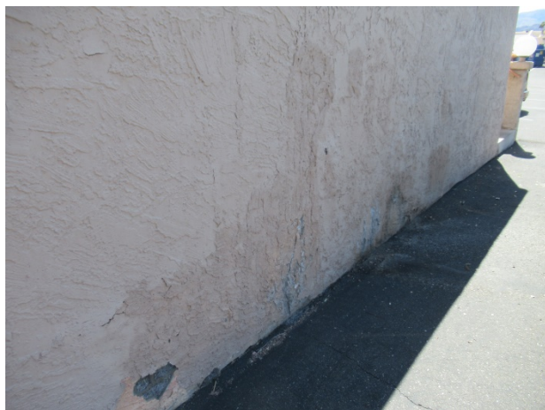
Stucco deterioration at retaining wall
