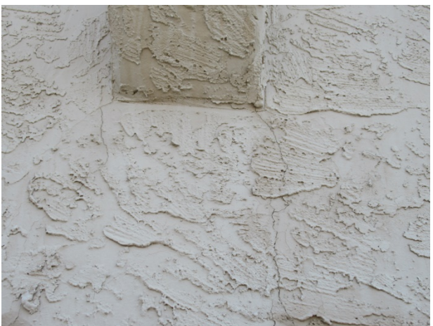
Stucco cracks
