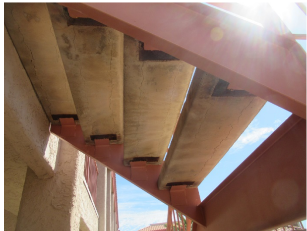
Tread cracks
