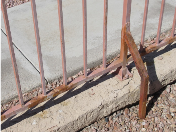
Area of corrosion at pool fence
