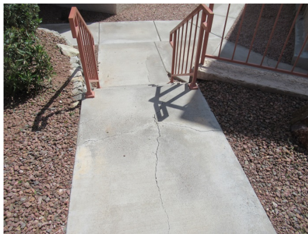
Sidewalk cracks
