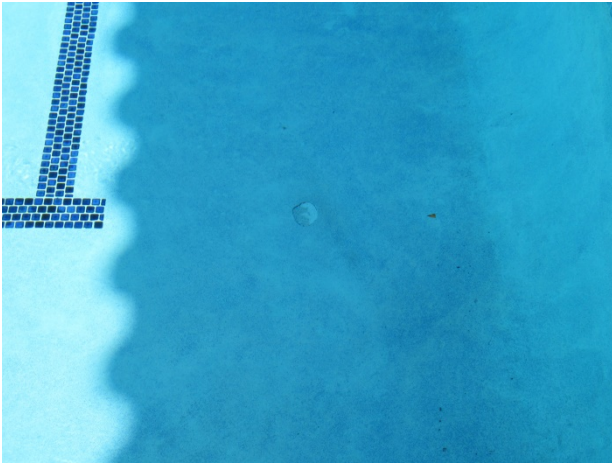
Chipped plaster at pool
