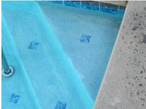
Chipped finish at pool step
