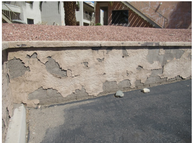
Significant coating deterioration east of the mailboxes
