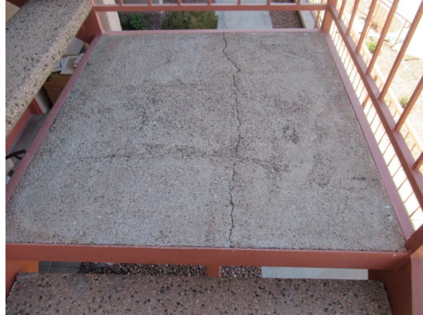
Cracks at concrete landing
