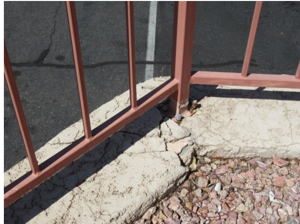
Retaining wall coping and fence post deterioration
