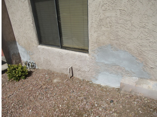
Repairs in progress
