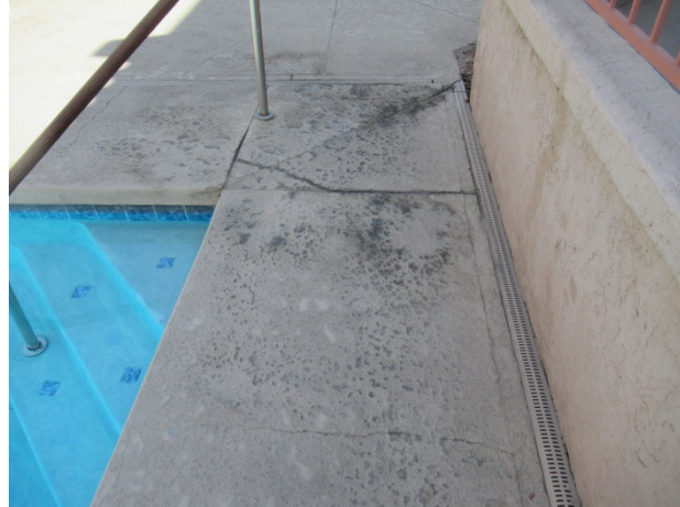
Minor cracks and coating deterioration
