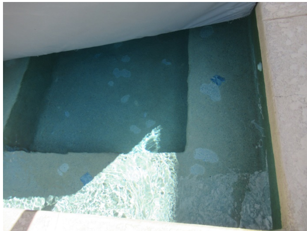
Chipped plaster at spa #2
