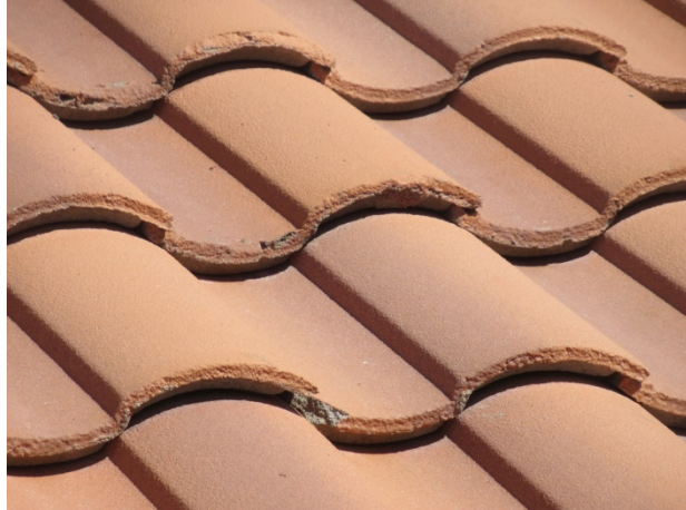
Minor chipped tiles
