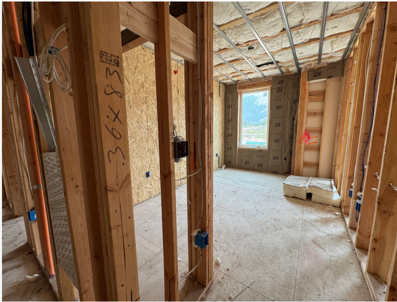
Interior work is advancing across multiple buildings
