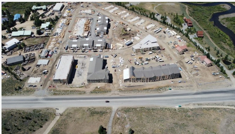
Site infrastructure continues alongside vertical construction
