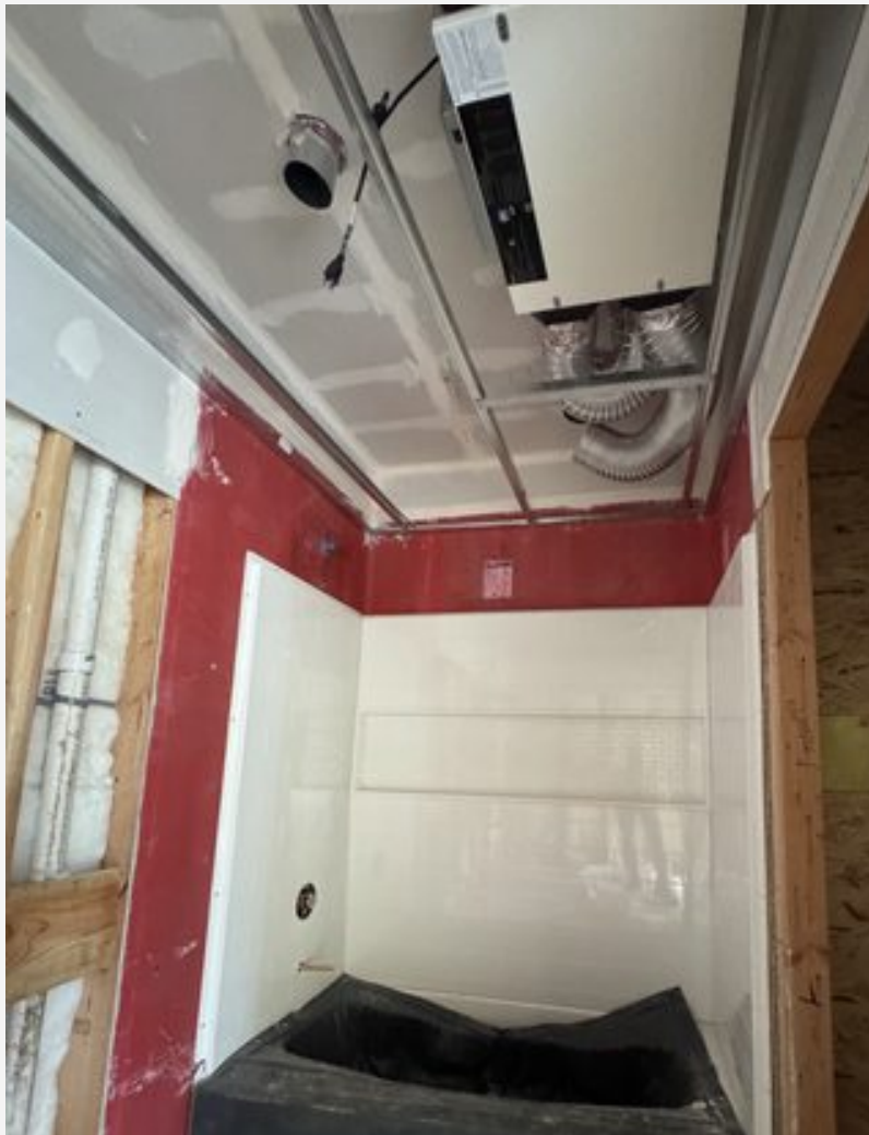
Drywall and trim progress show homes moving closer to finish
